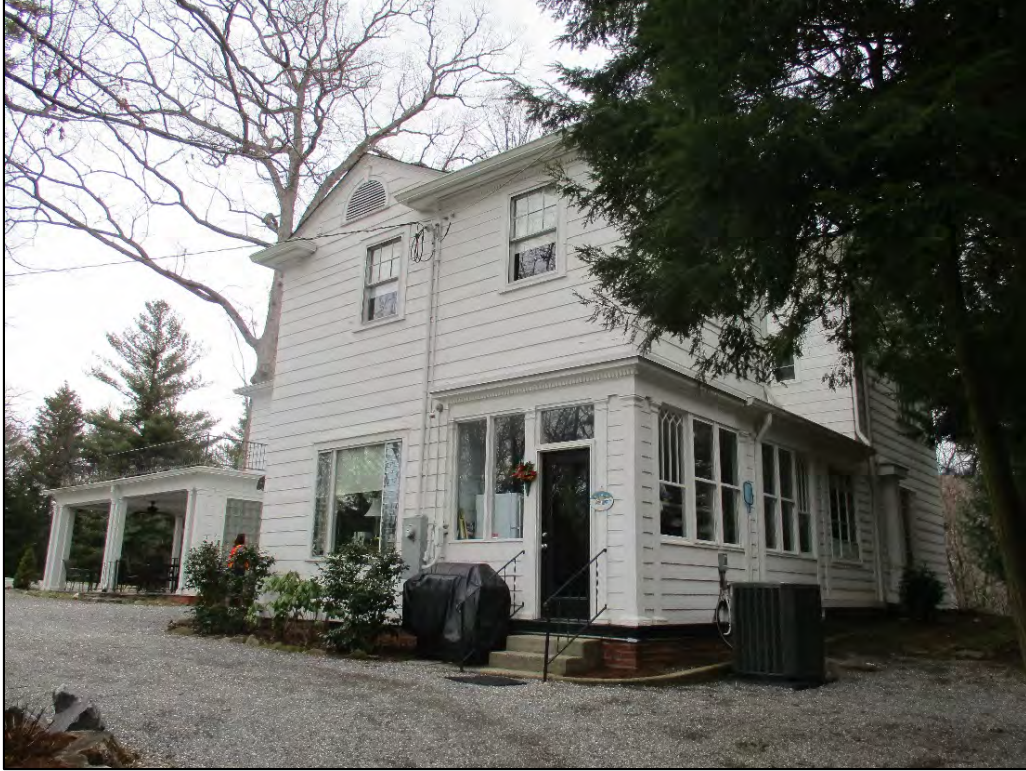
Rhodes House rear (west) elevation, view to the northeast
