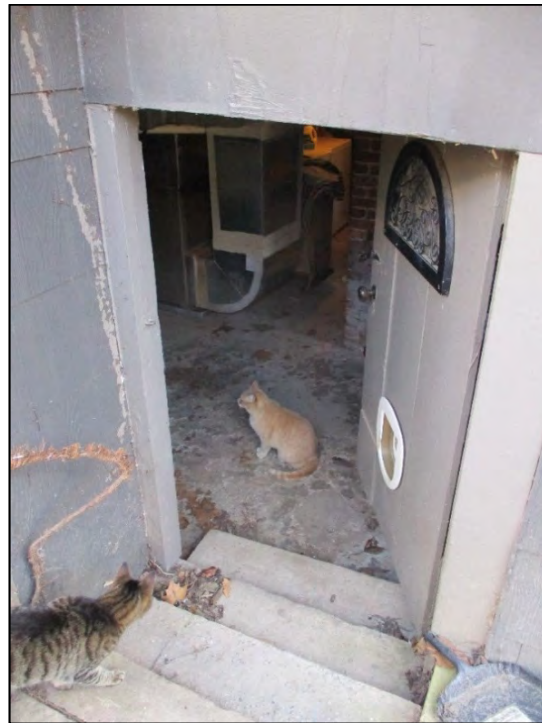
Weaver House north elevation basement entrance
