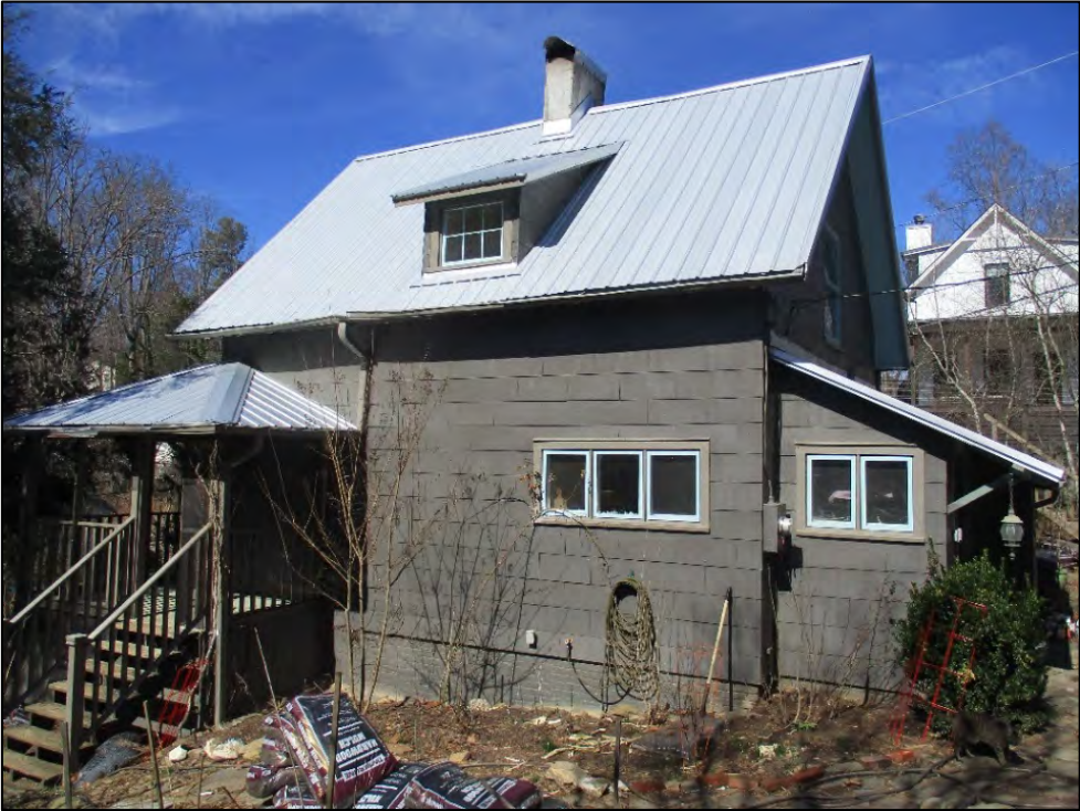
Weaver House south elevation, view to the north
