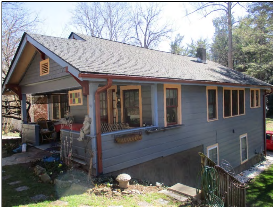
Williams House oblique view of façade and west elevation, view to the southeast
