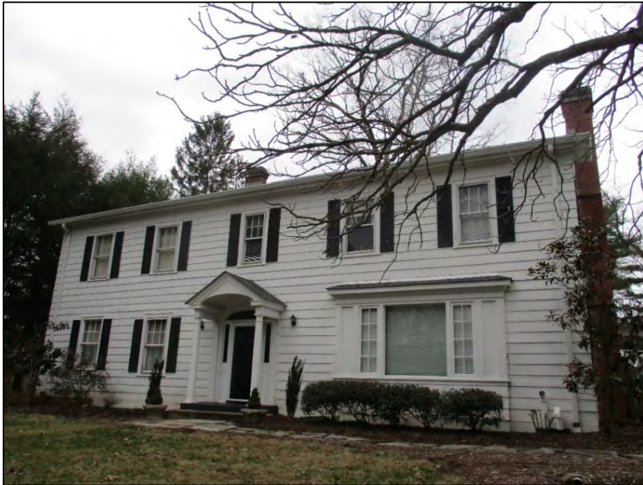
Rhoades House façade, view to the west
