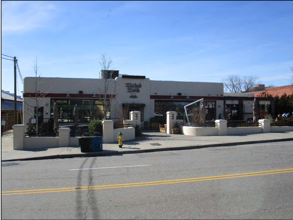
Exhibit 126. GulfPride Service Station (BN5180) (1941), 91 Biltmore Avenue in Downtown Asheville Historic District Boundary Increase IIIb
