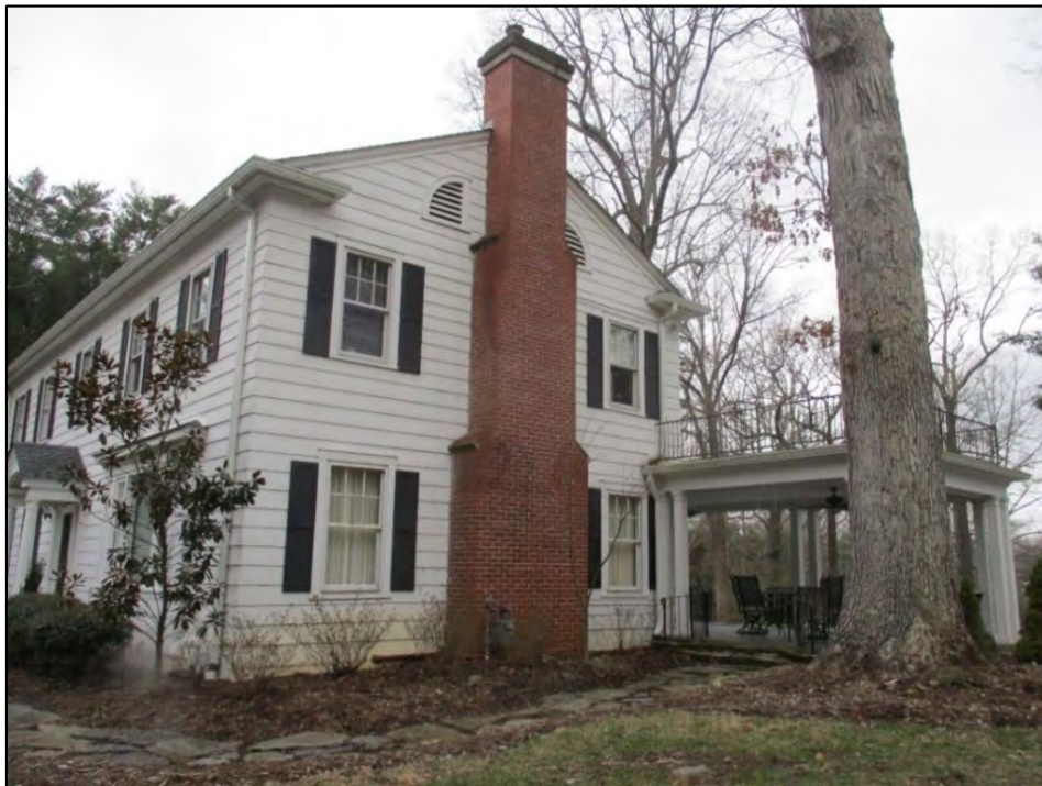
Rhoades House north elevation, view to the southwest
