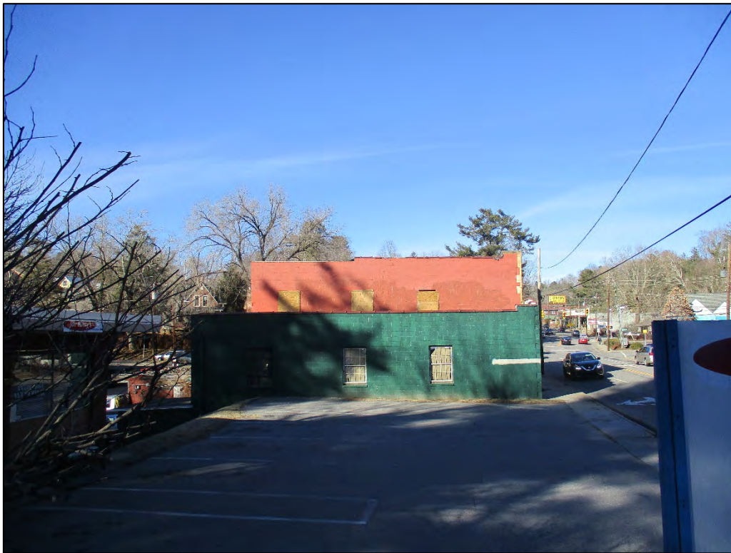
Former Moser Plumbing Building south elevation, view to the north. Keith's Super-Cleaners is in foreground.
