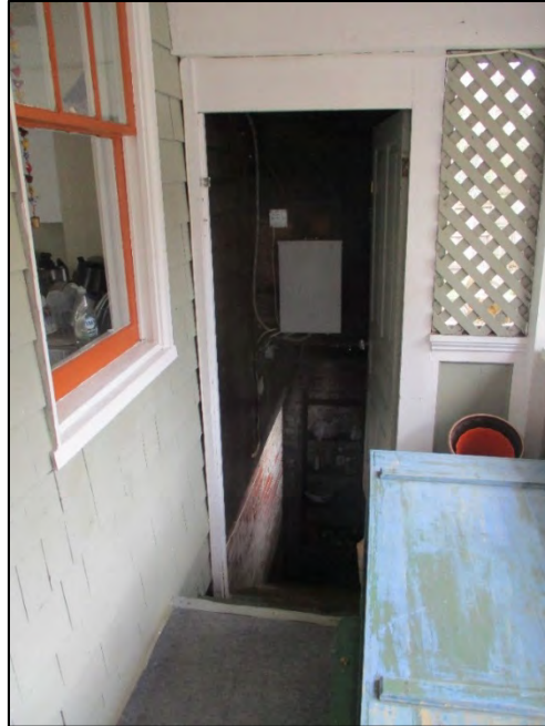
Lauerhass House rear porch detail and view into basement
