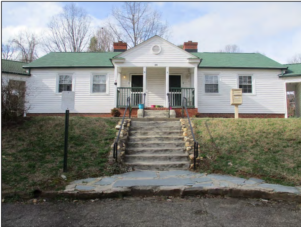
Clearview Terrace Apartments Building A, Units 2 and 3 façade, view to north
