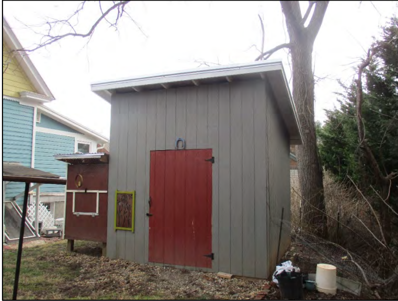
Barber House outbuilding with attached chicken coop, view to the southeast
