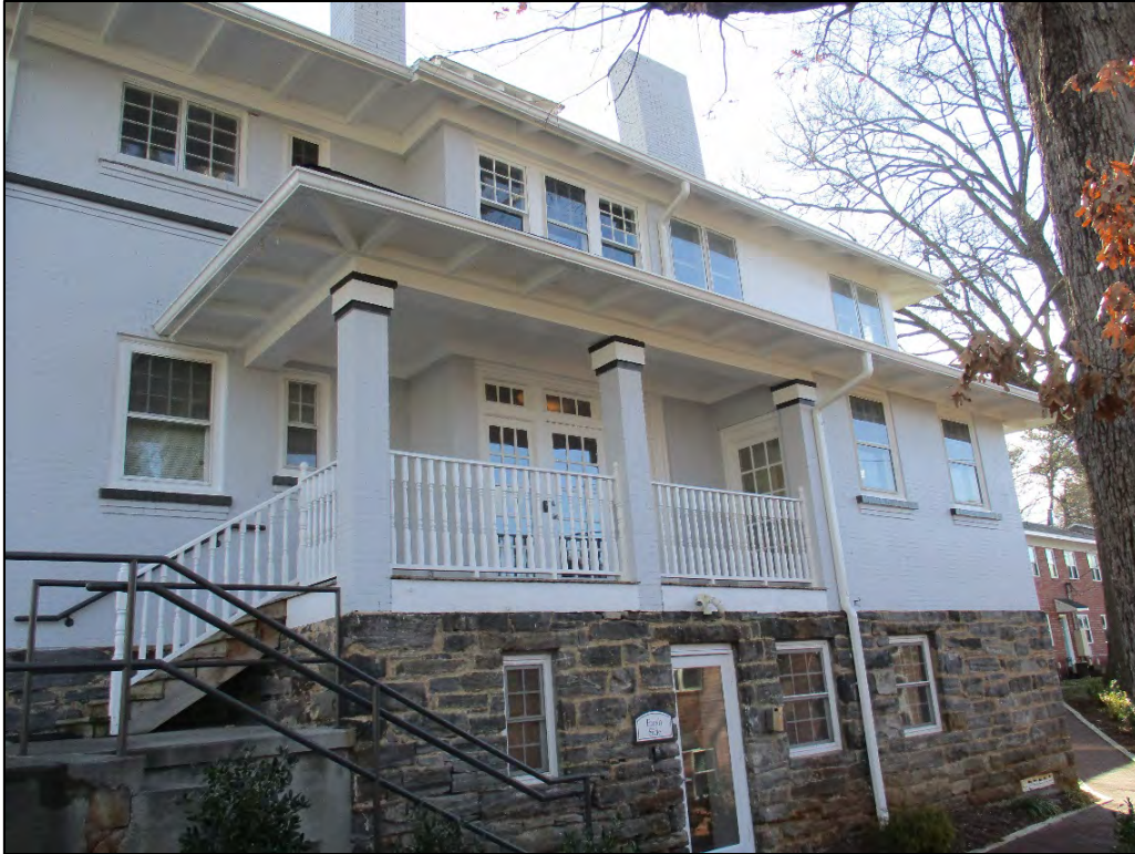
Edgewood Knoll Apartments leasing office west elevation, view to southeast
