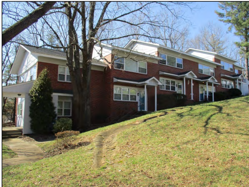
Edgewood Knoll Apartments Building 3 primary elevation, view to southwest
