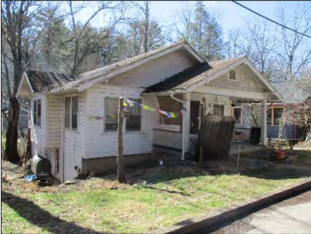
Atkins House elevation view to the southwest
