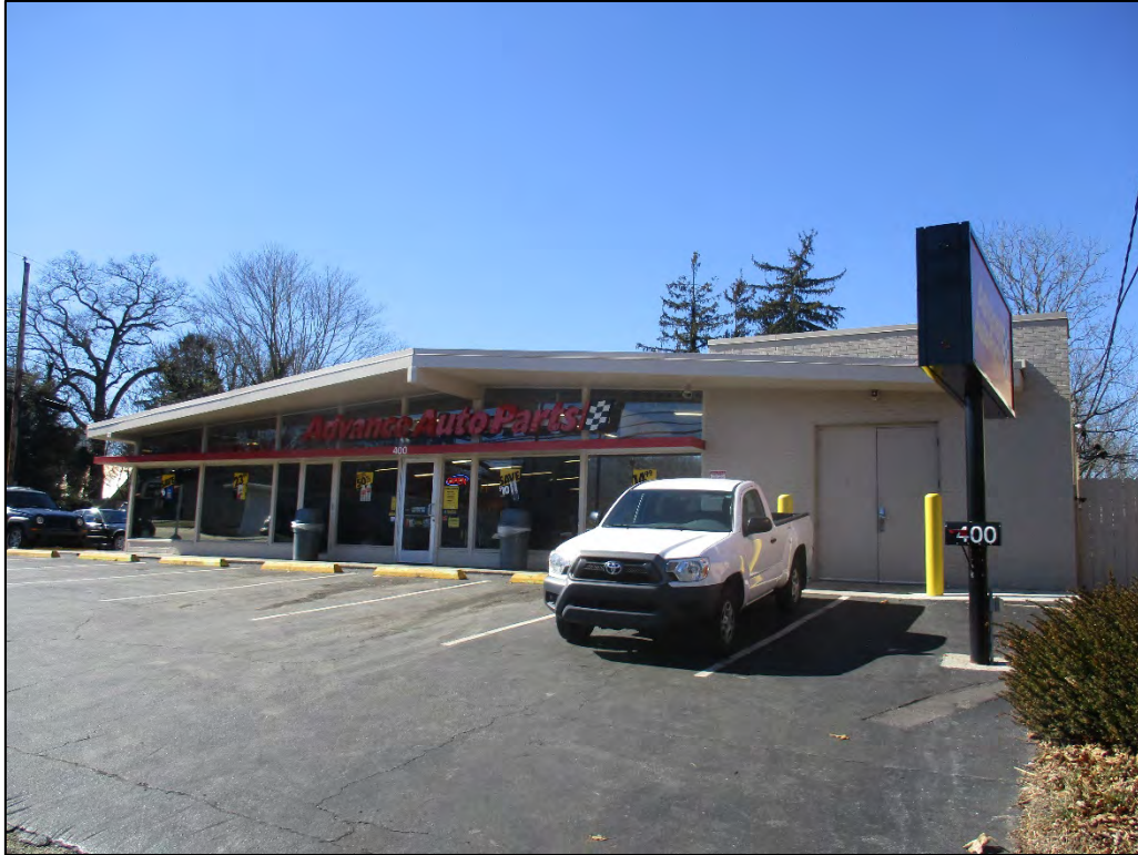
Former Glidden Drive-In Paint Center façade, view to the southwest
