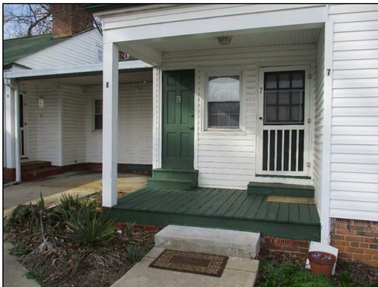
Clearview Terrace Apartments Building B, Unit 7 and 8 façade, porch detail
