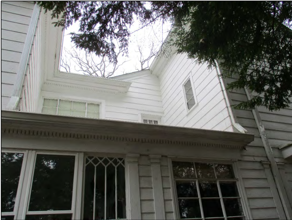
Rhoades House south elevation, second-story detail
