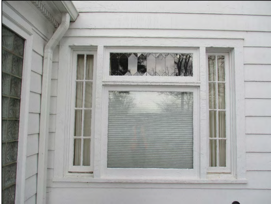
Rhoades House rear (west) elevation picture window detail
