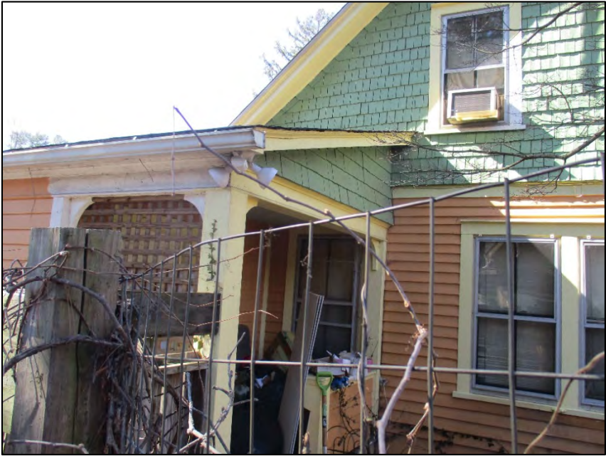
Guischard House east elevation, view to the west
