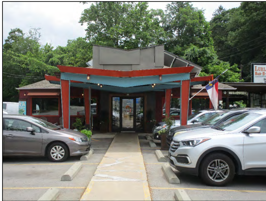
Former A&W Drive-In façade, view to south
