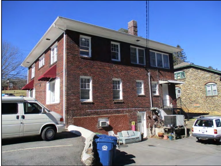
Rear (east) elevation, view to the northwest
