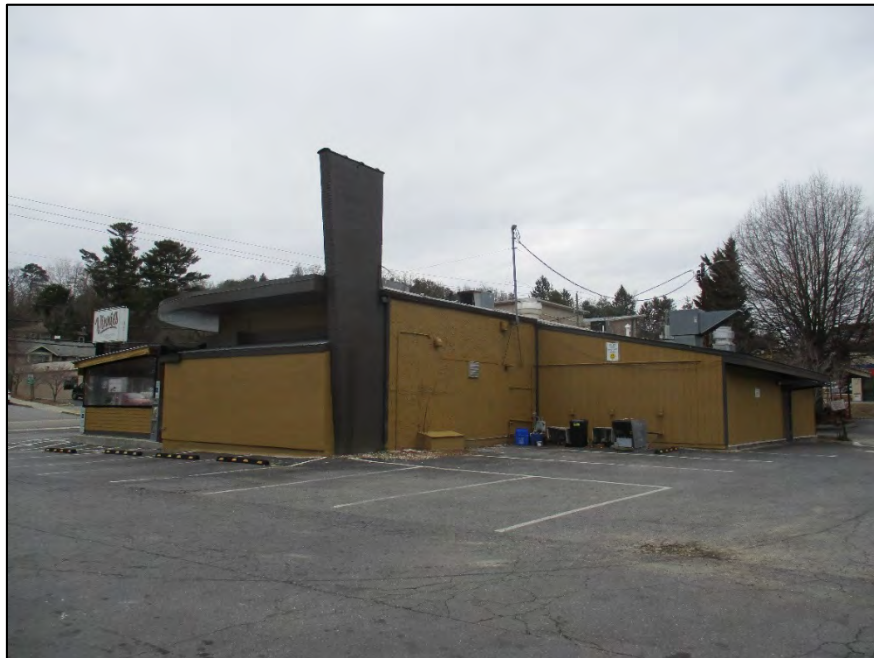
Former Athens Restaurant oblique view of south and rear (east) elevations, view to northwest
