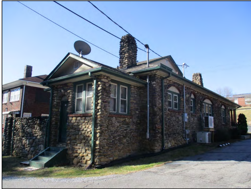
Former Belva L. Saunders House oblique view of north and east (rear) elevations, looking southwest
