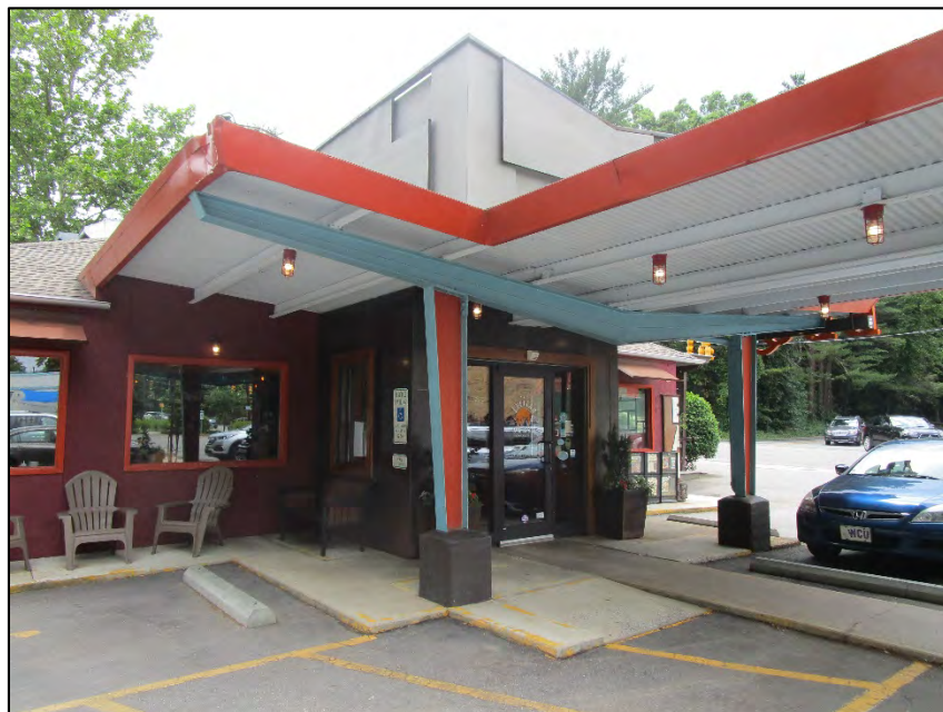
Former A&W Drive-In façade, canopy detail, view to southwest
