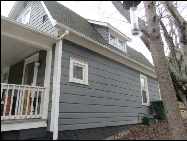
Joseph Lewis House north elevation, view to the southwest
