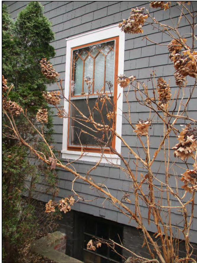
North elevation window detail
