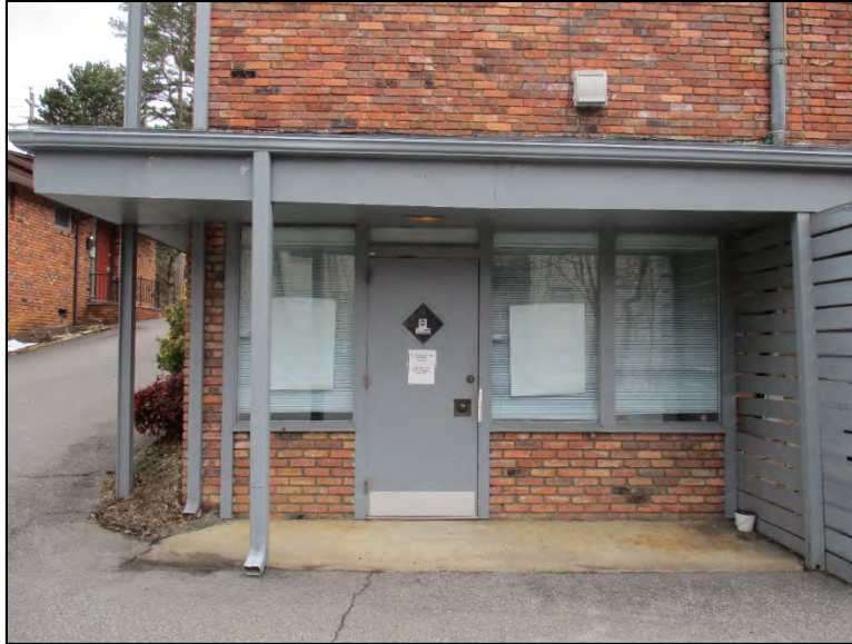
Thompson Building rear (east) elevation entry detail, looking west
