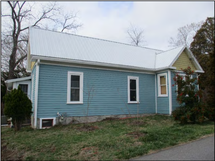
Barber House east elevation, view to northwest
