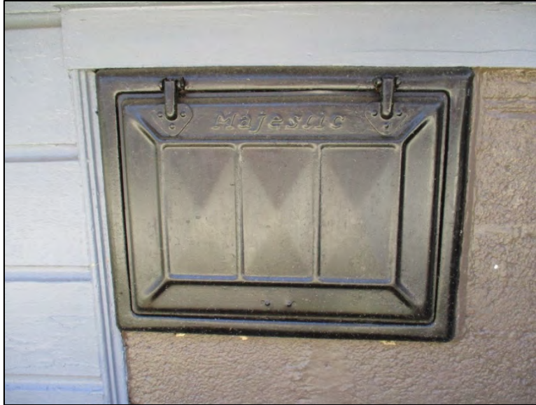
Williams House east elevation, coal chute detail
