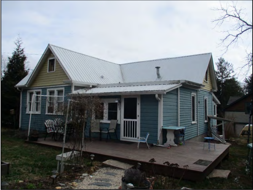
Barber House north elevation, view to southeast
