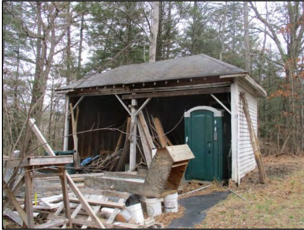
Rhoades House storage shed west elevation, view to the east
