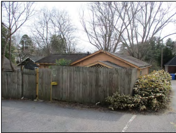
Lauerhass House outbuilding façade from alley, view to the south
