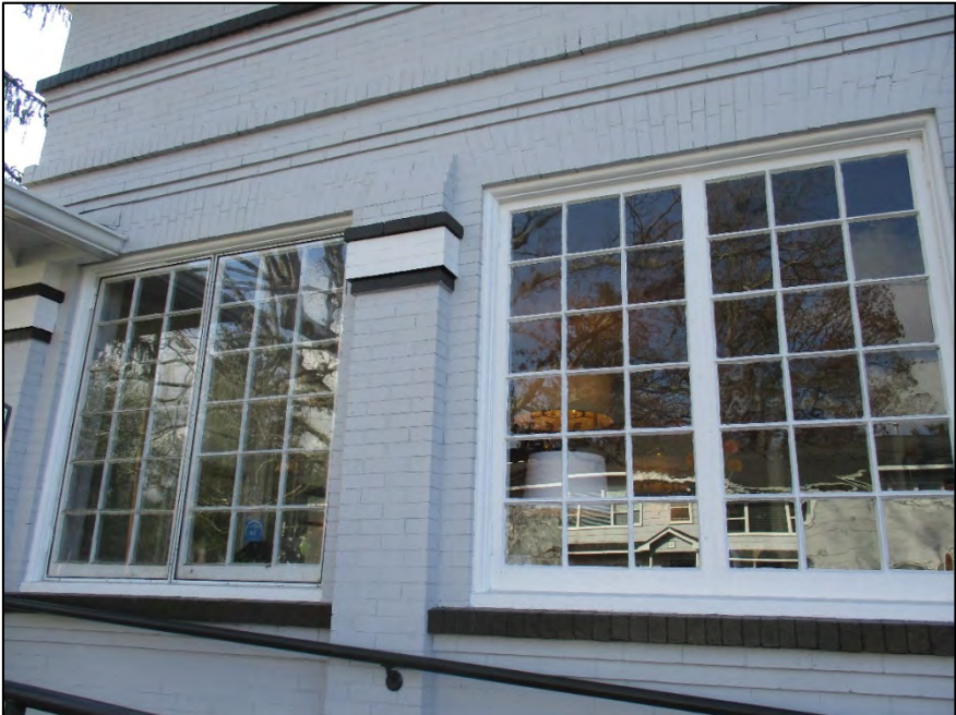
Edgewood Knoll Apartments leasing office north elevation window detail
