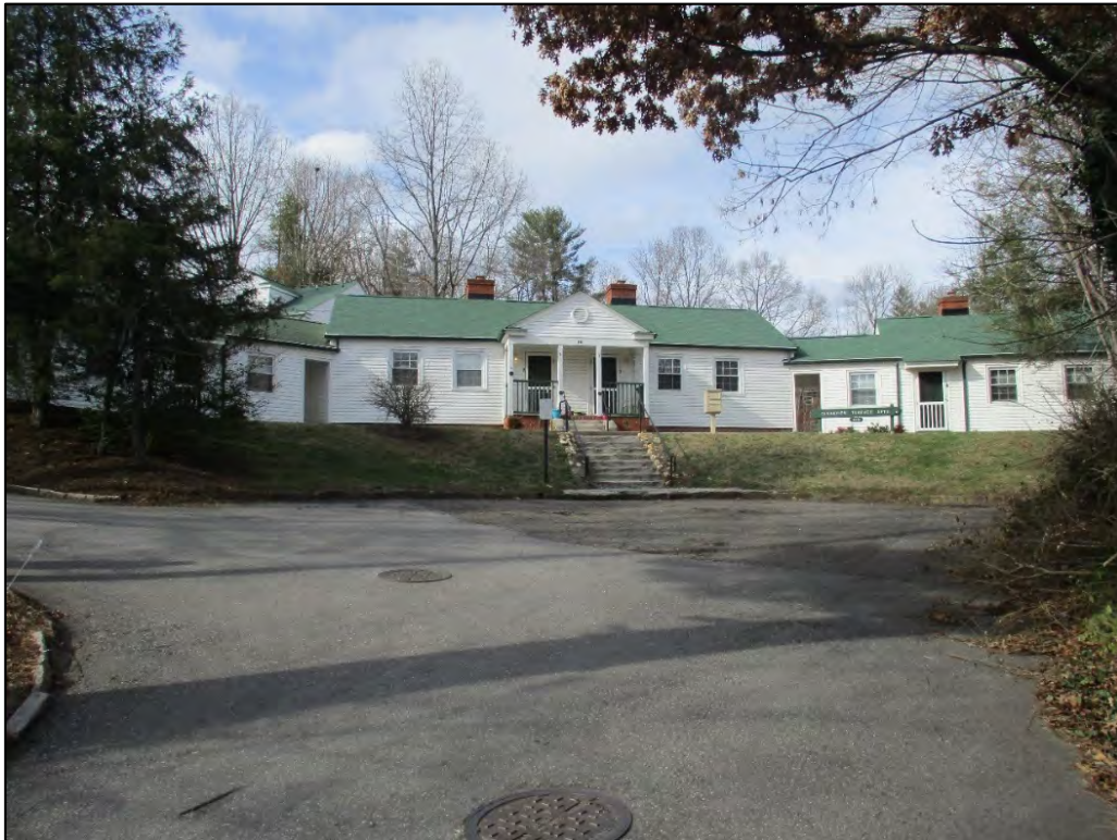
Clearview Terrace Apartments Building A façade, view to north
