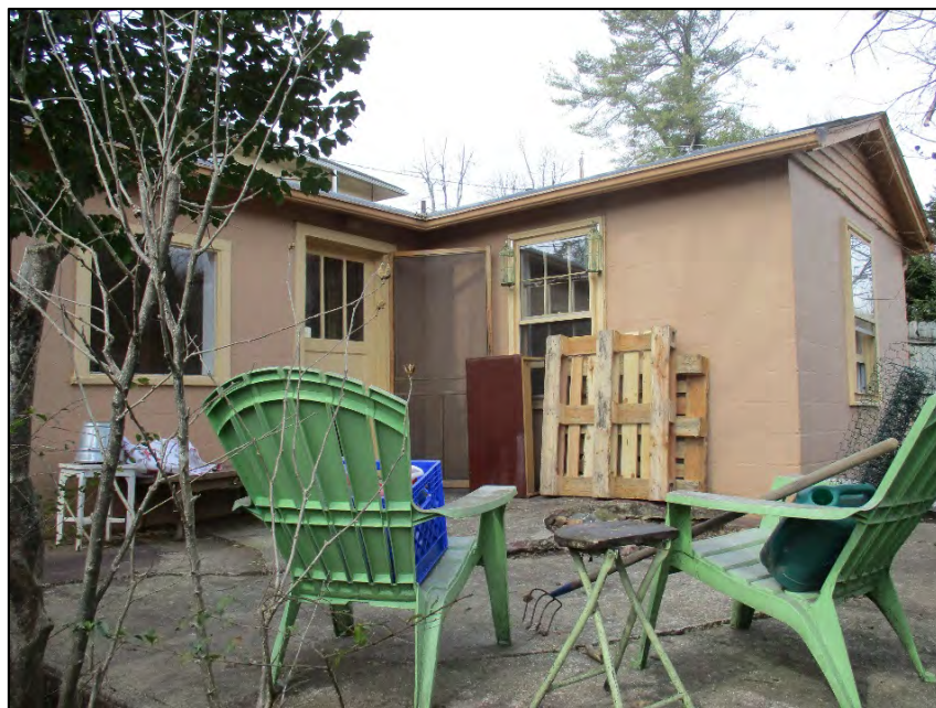
Lauerhass House outbuilding rear elevation view to the northwest
