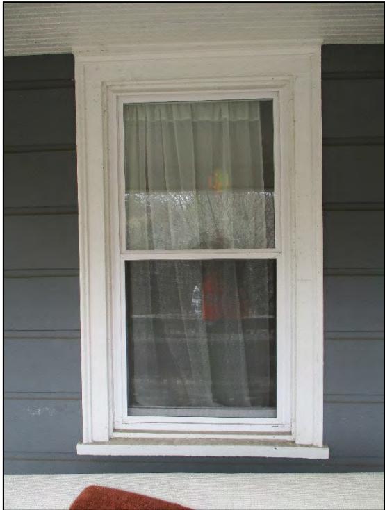
Joseph Lewis House front porch window detail
