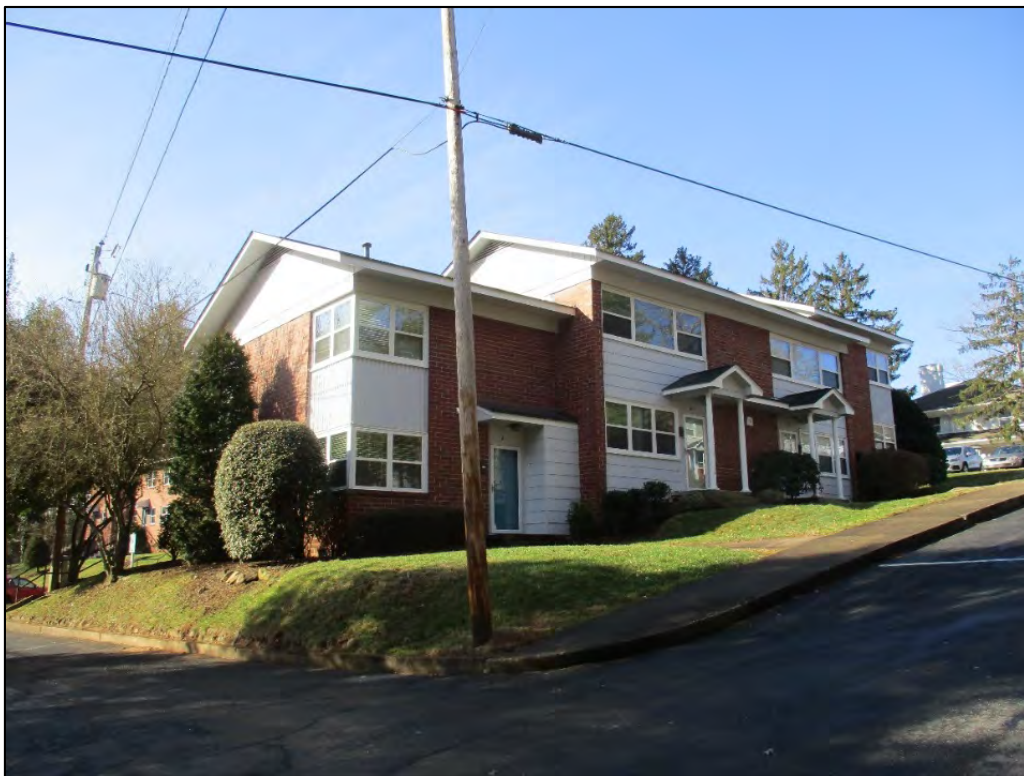
Edgewood Knoll Apartments Building 10 façade, view to the southwest
