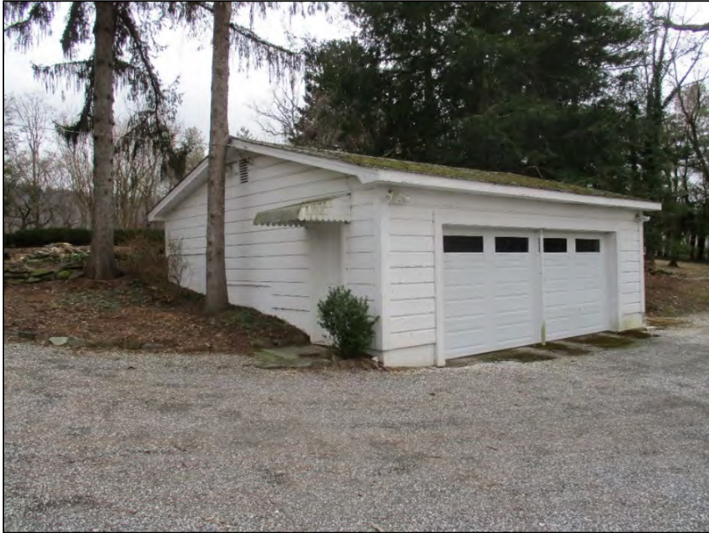
Rhoades House garage, view to the southeast
