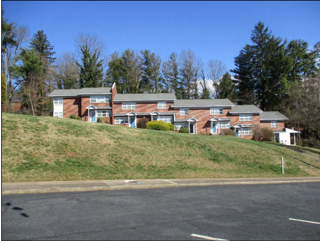
Edgewood Knoll Apartments Building 2 façade, view to north
