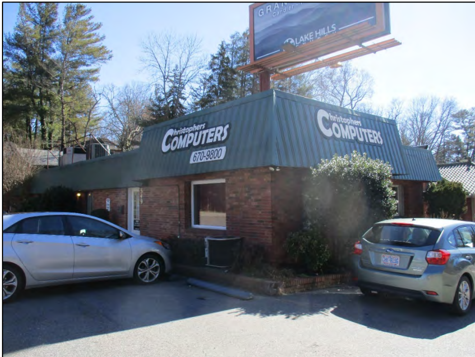
Farrwood Tourist Court oblique view of northwest corner – likely motel office – view to the southeast
