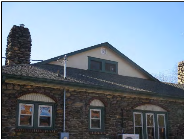
Former Belva L. Saunders House north elevation gable detail, facing southwest
