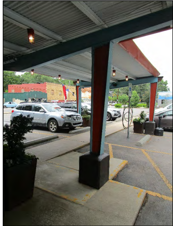
Former A&W Drive-In, canopy detail, view to northwest
