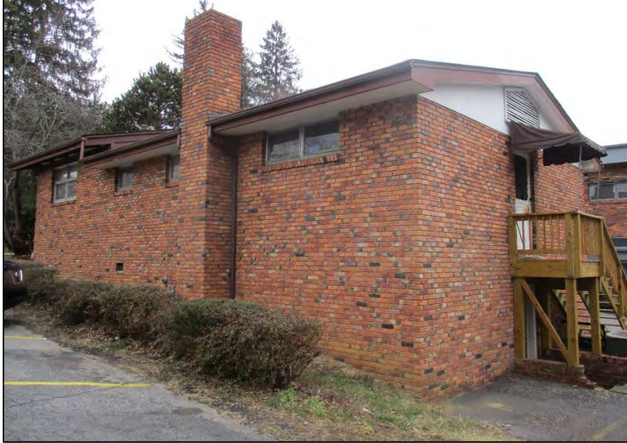
Ray Dental Office oblique view of south and rear (east) elevations, looking northwest
