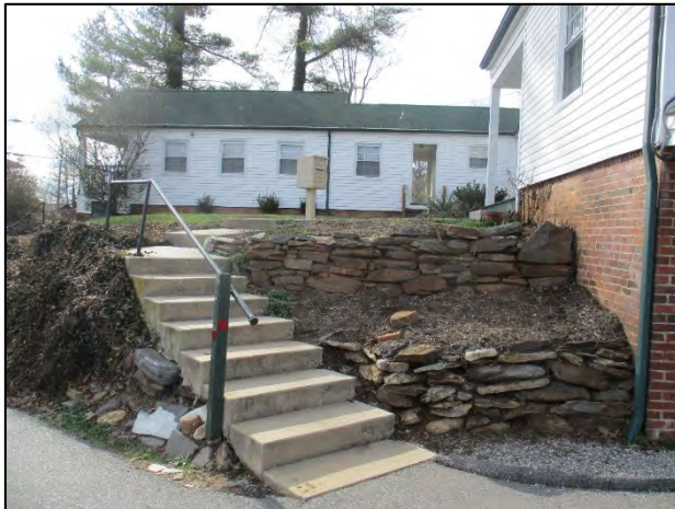
Clearview Terrace Apartments Building B landscaping detail, view to west
