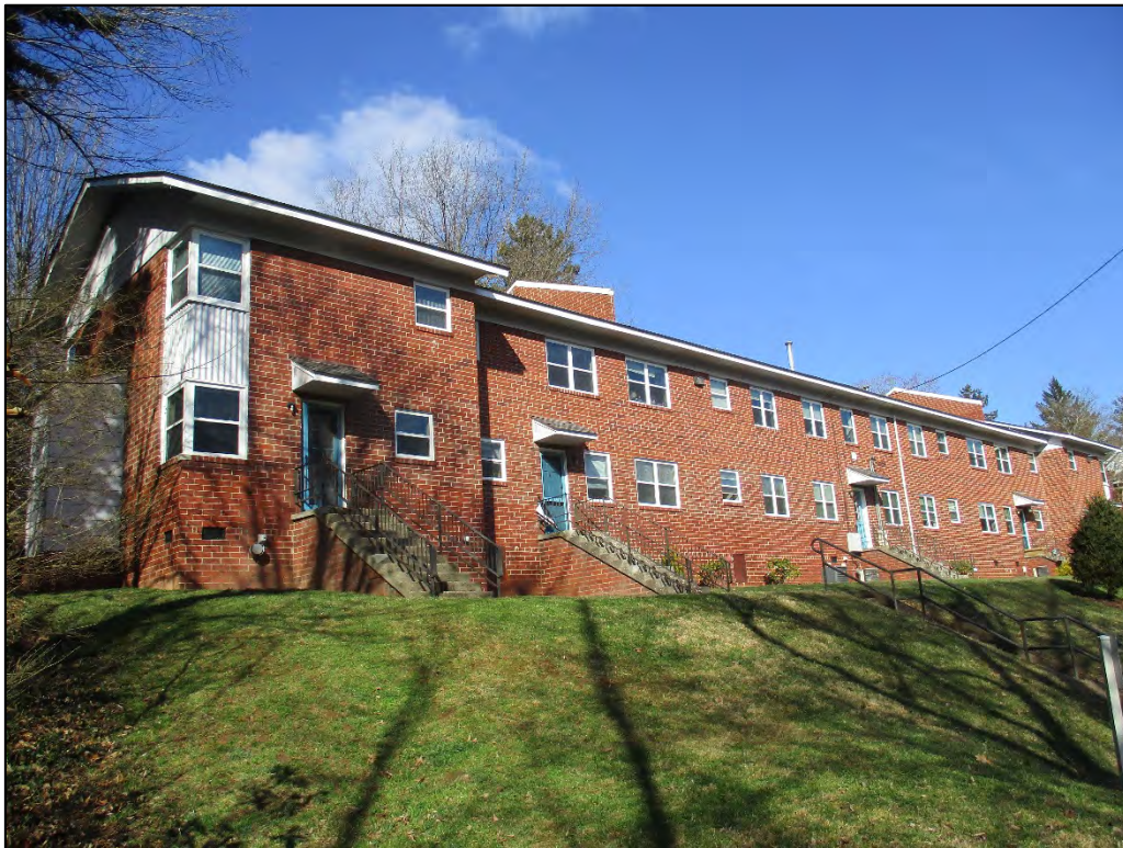
Edgewood Knoll Apartments Building 9 rear (east) elevation, view to southeast
