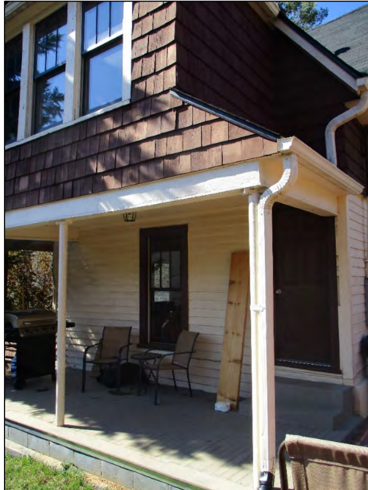
Martha Sayre House east elevation engaged porch detail
