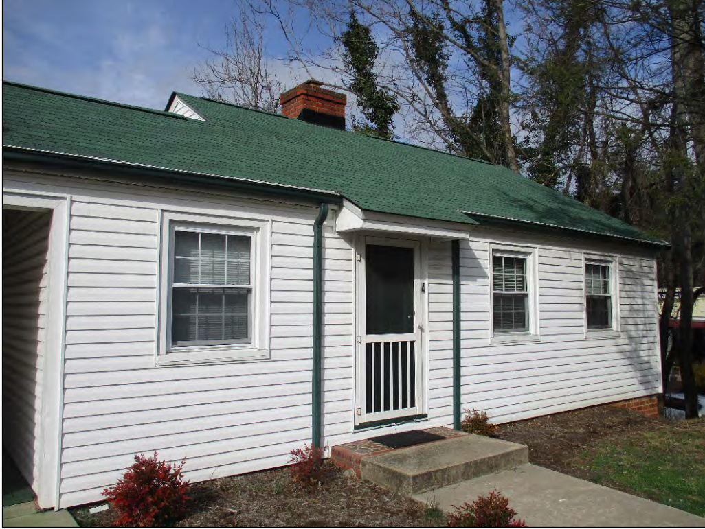
Clearview Terrace Apartments Building A, Unit 4 façade, view to northeast
