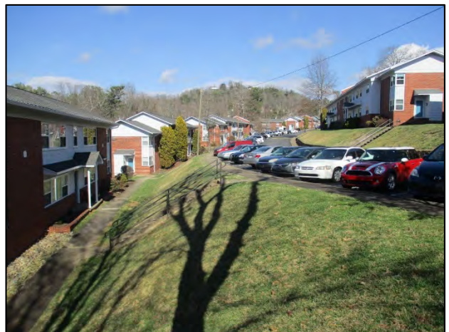
Edgewood Knoll Apartments, view to the north of Edgewood Knoll Road from outbuilding/garage
