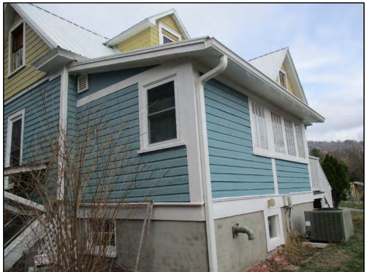
Barber House oblique view of façade, enclosed porch, and west elevation, view to northeast
