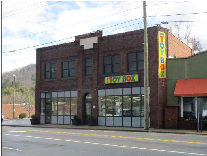
Exhibit 30. Robinson Building (BN5749) (1927), 793 Merrimon Avenue
