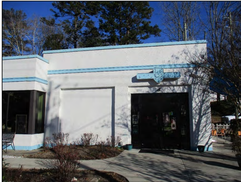
Former Woolsey Dip Amoco Station façade service bay detail, view to east. One service bay door is infilled at left, the other converted to a secondary entry.
