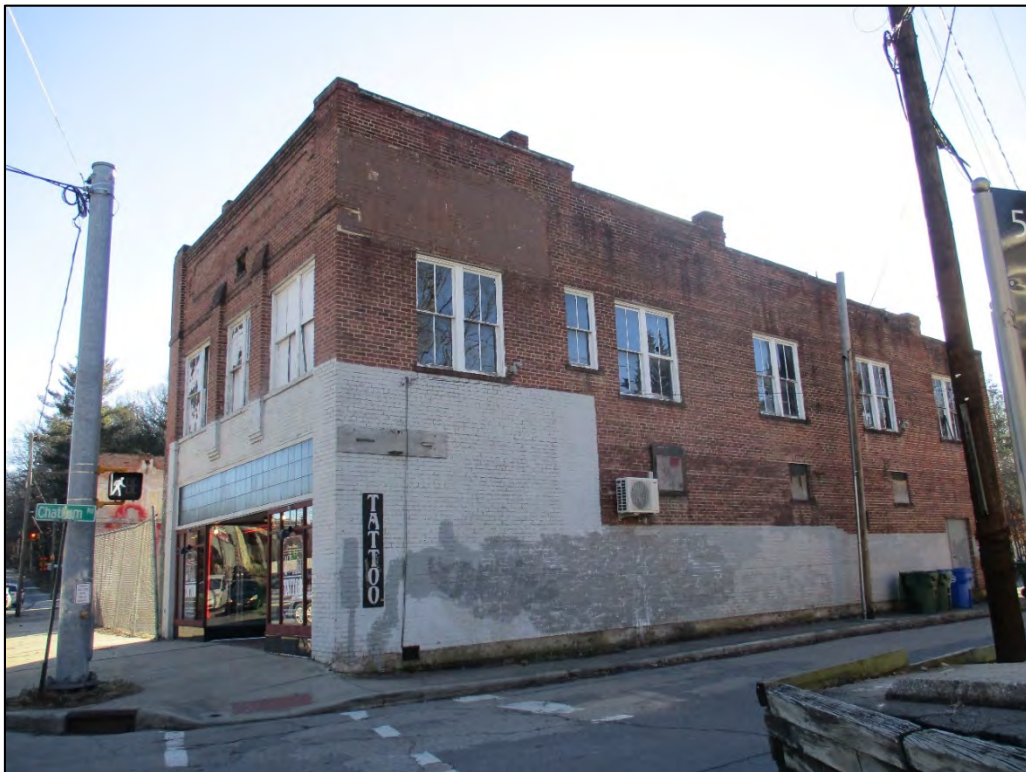
Allison's Grocery oblique view of the façade (east facing) and north elevation, looking to the southwest
