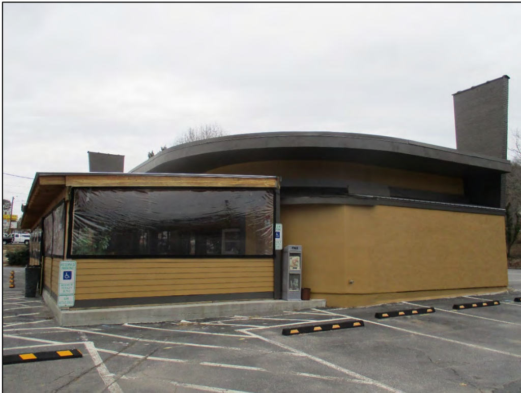
Former Athens Restaurant south elevation, view to north
