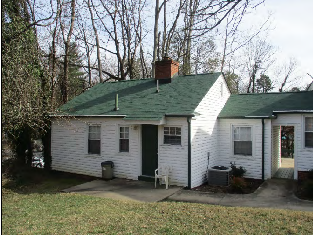
Clearview Terrace Apartments Building A, Unit 4 rear (north) elevation, view to southeast
