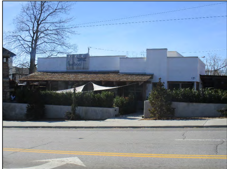
Exhibit 125. O’Kelley’s Amoco Service Station (BN5182) (1944), 121 Biltmore Avenue in Downtown Asheville Historic District Boundary Increase IIIb
