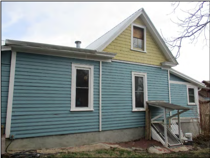
Barber House west elevation, view to southeast
