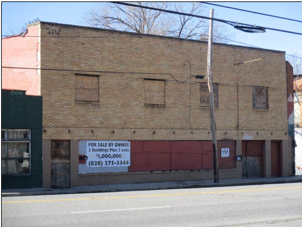
Former Moser Plumbing Building façade, view to the northwest
