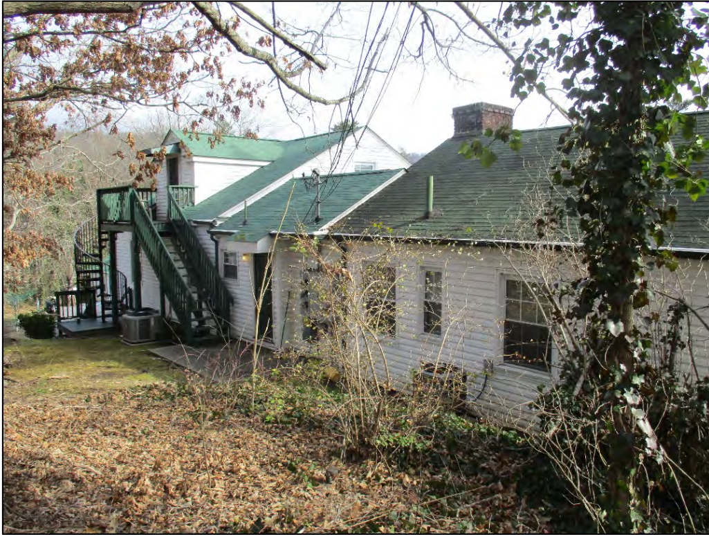
Clearview Terrace Apartments Building B, Units 6, 7, and 8 rear (north) elevation, view to southeast
