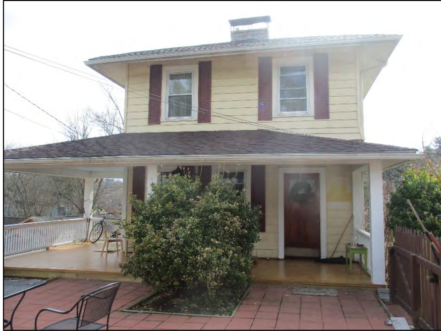
Façade, view to the south
