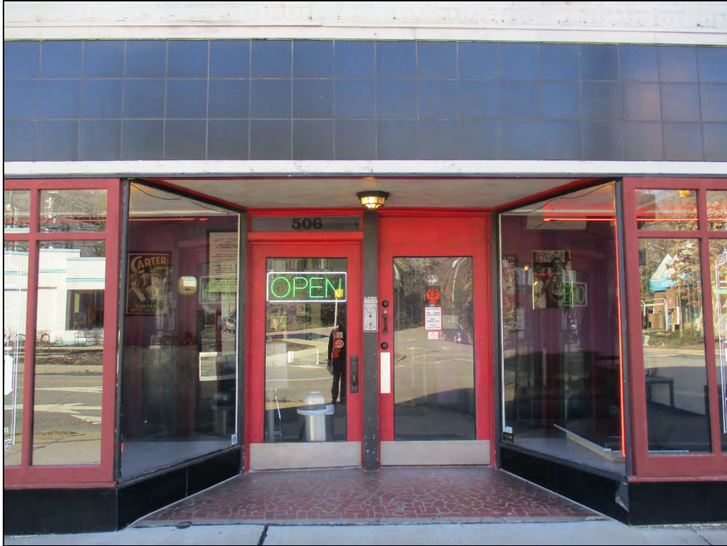
Allison's Grocery façade entry detail, facing west
