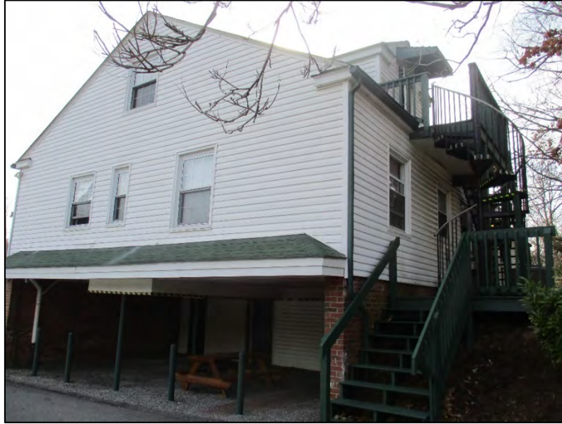
Clearview Terrace Apartments Building B, Units 7 and 8 east elevation over converted carport/garage, view to southwest
