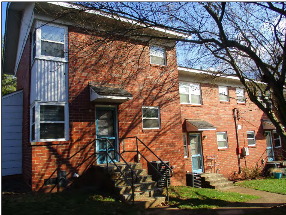
Edgewood Knoll Apartments Building 10 rear (south) elevation, view to northeast
