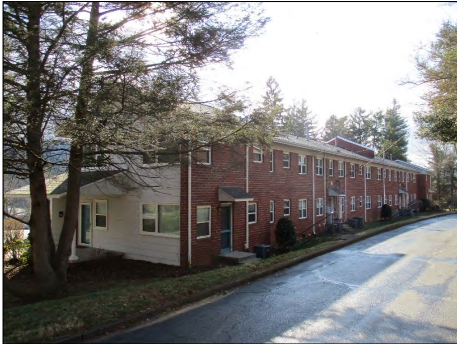
Edgewood Knoll Apartments Building 11 rear (west) elevation, view to southeast
