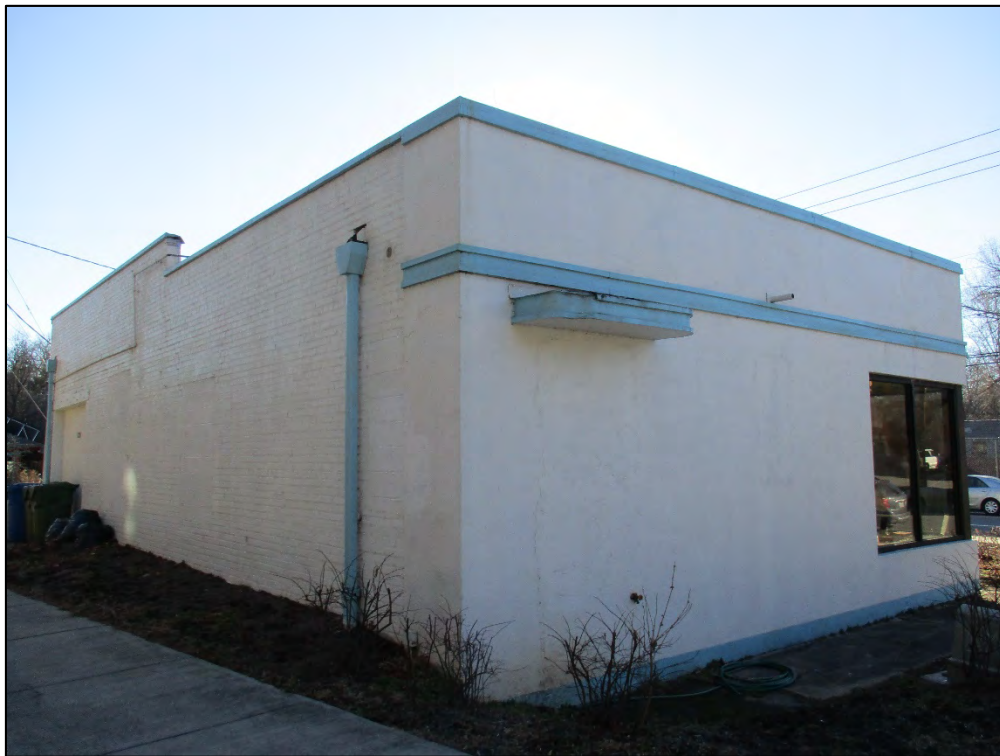
Former Woolsey Dip Amoco Station oblique view of the north and rear (east) elevations, view to the southwest. Note hood above the infilled bathroom door in rear of north elevation.
