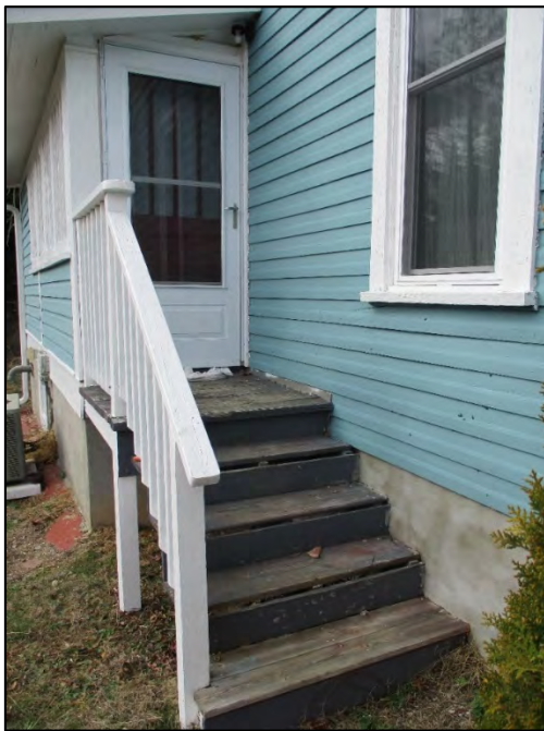
Barber House former front door on south elevation, view to northwest
