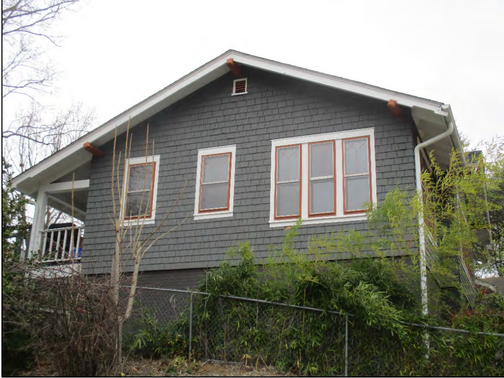
South elevation, view to the north
