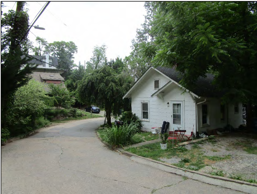
24 Chatham Road (1927), view to the southeast
