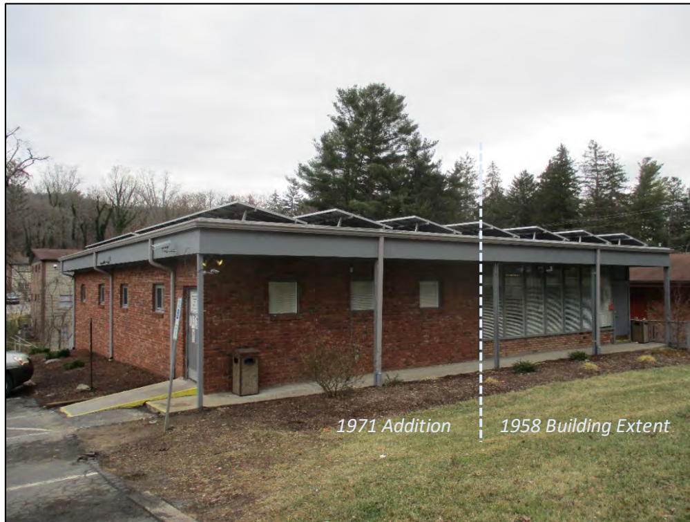
Thompson Building oblique view of the façade and north elevation, view to the southeast
