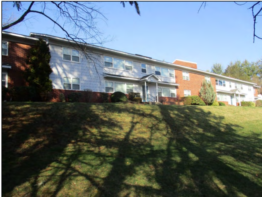
Edgewood Knoll Apartments Building 11 façade, view to northwest
