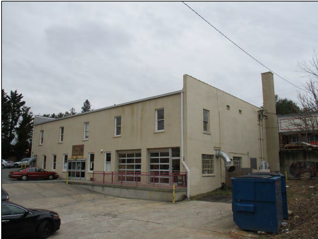
Oblique view to the southwest of Burton and Son Furniture Store north elevation and rear (east) elevation
