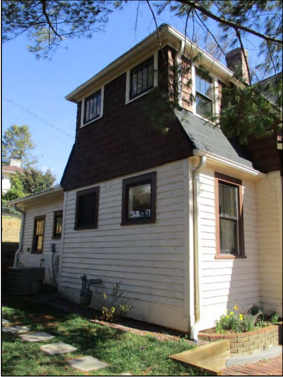
Martha Sayre House west elevation, view to the northeast
