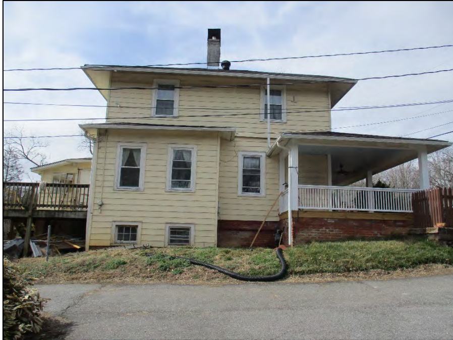
East elevation view to east
