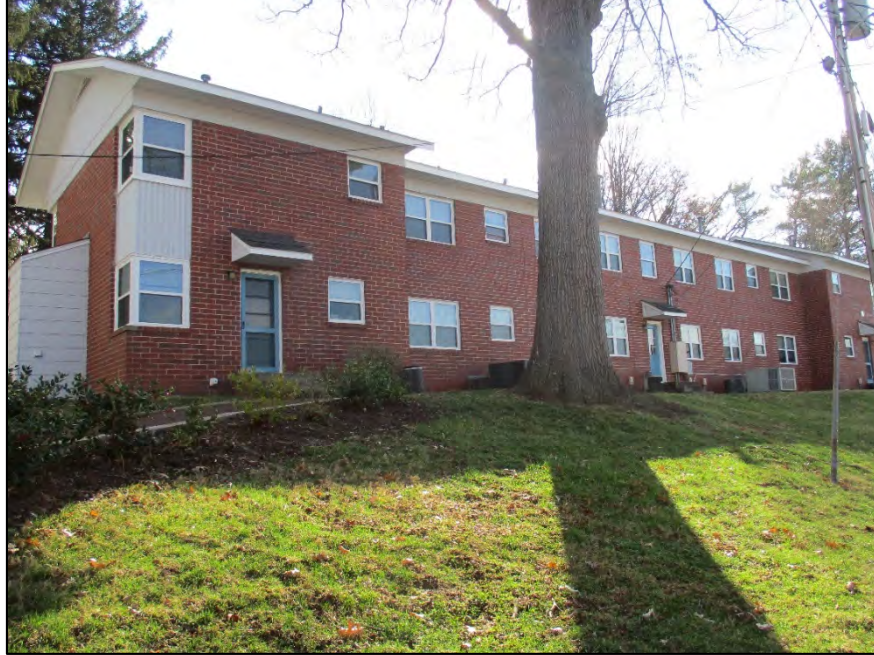
Edgewood Knoll Apartments Building 7 rear elevation, view to southeast
