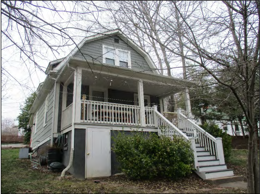
Joseph Lewis House oblique view of façade and south elevation, view to the northwest
