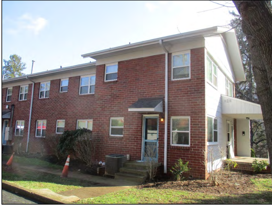
Edgewood Knoll Apartments Building 11 rear (west) elevation, view to east
