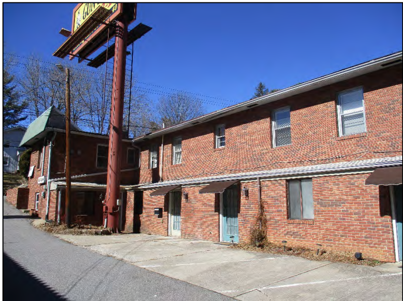
Farrwood Tourist Court south elevation, view to the northwest
