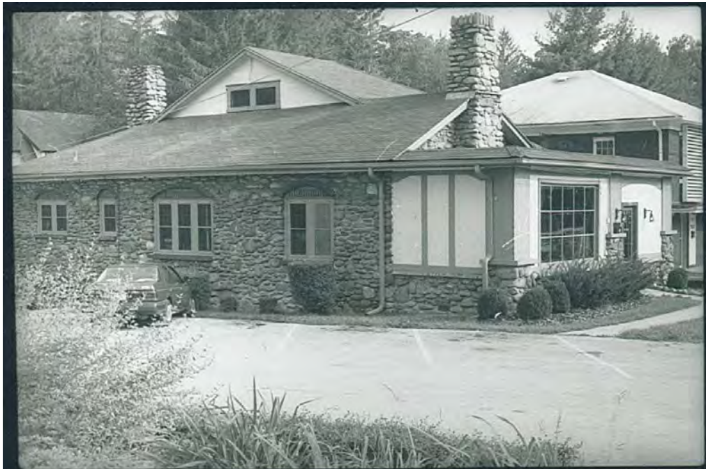
Exhibit 109. The (former) Belva L. Saunders House at the time of the 1989 survey. Note the six-over-one windows in the north elevation. Credit: Mary Hooper, 1989.
