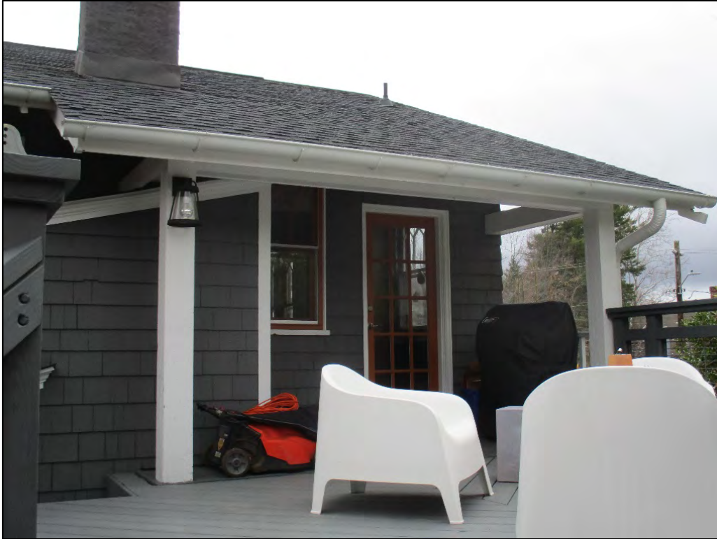
West elevation porch detail
