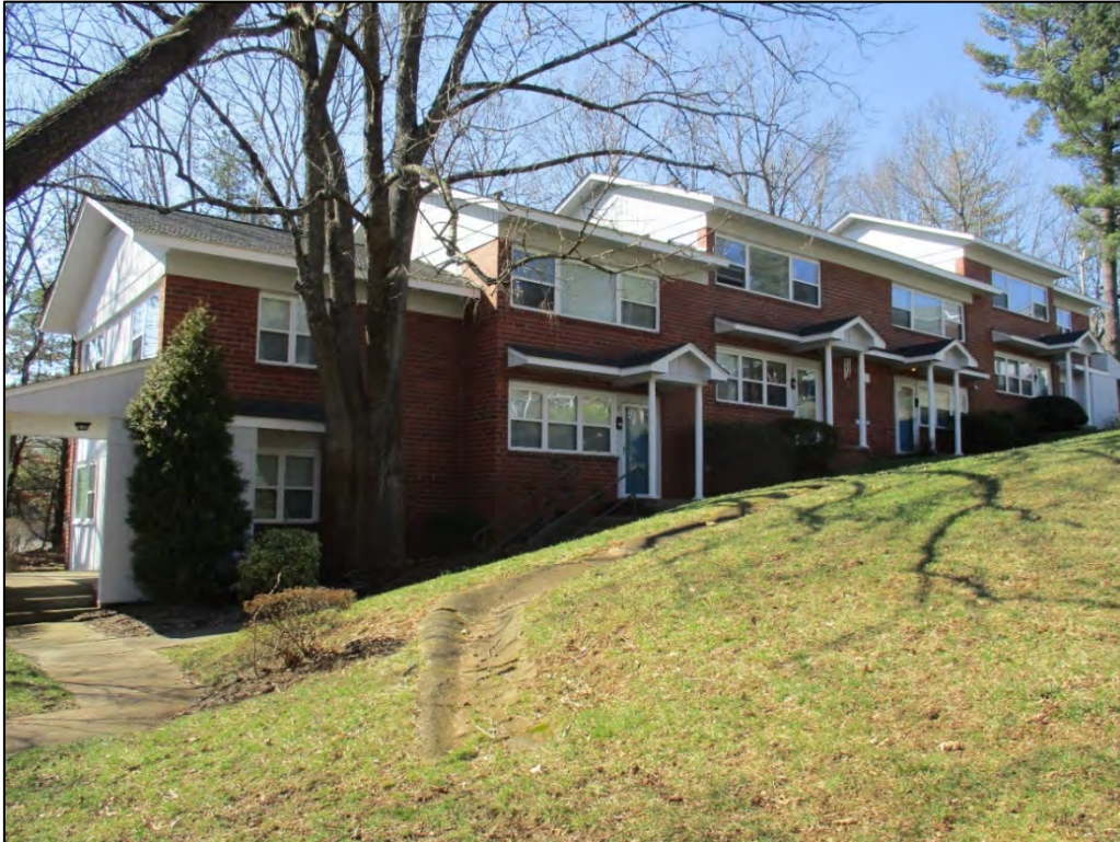
Edgewood Knoll Apartments, Building 3 façade, view to northwest
