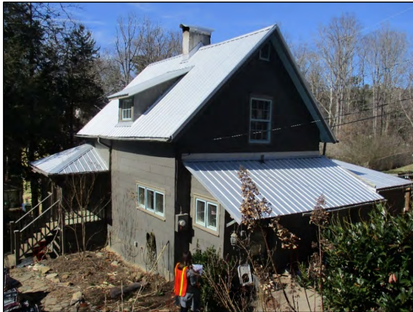
Weaver House east elevation, view to the northwest
