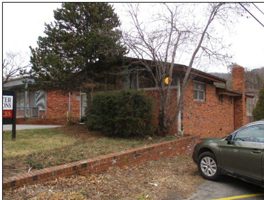
Ray Dental Office oblique view of façade and south elevation, looking northeast
