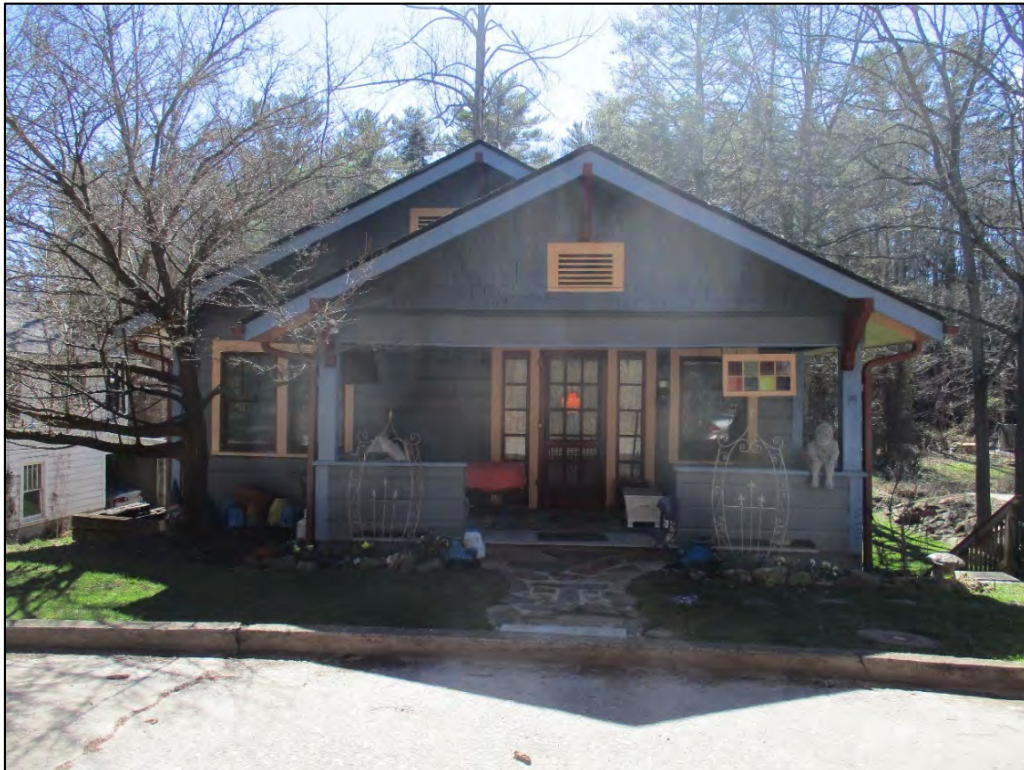
Williams House façade, view to the south
