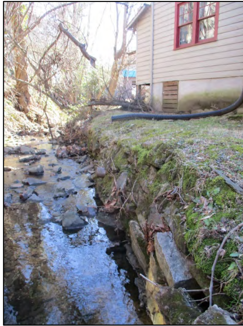
View along unnamed creek at east parcel boundary. Note laid stone embankment and proximity of house at right.
