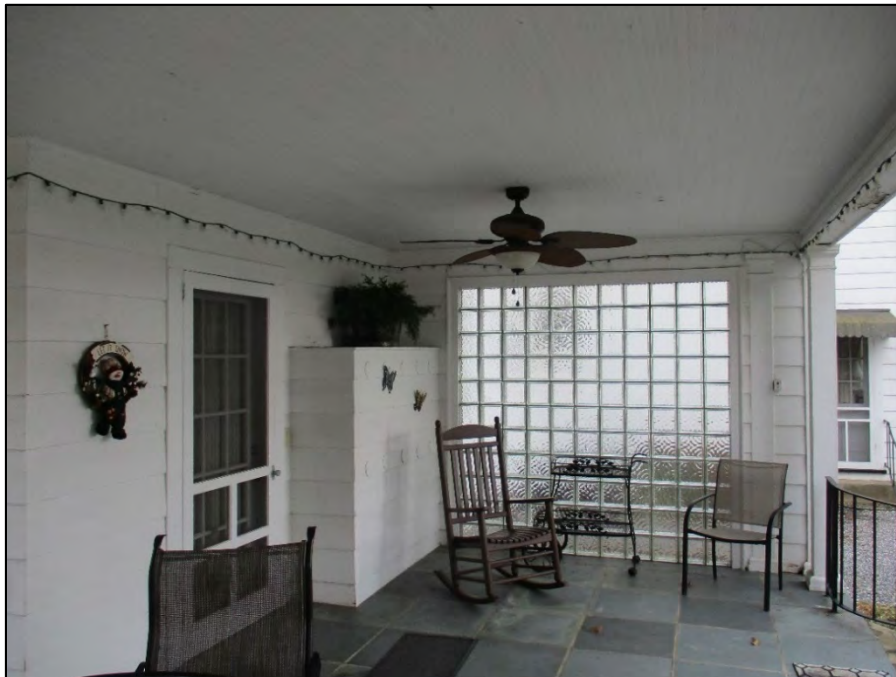
Rhoades House rear (west) elevation porch detail, view to the south
