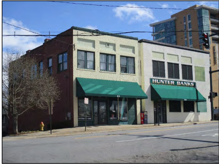
Exhibit 31. Commercial Building (BN2802) (1923), 31 Montford Avenue (at left) in the Montford Area Historic District
