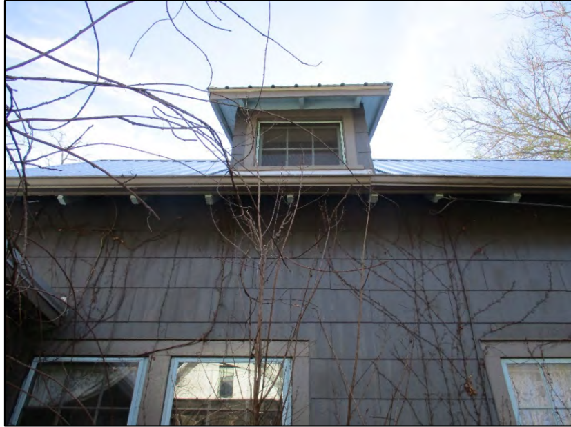
Weaver House north elevation shed dormer, view to the south
