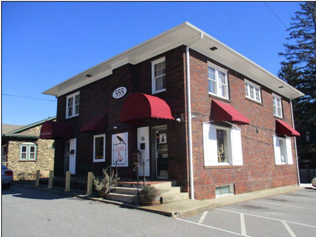
Oblique view of façade and south elevation, view to the northeast
