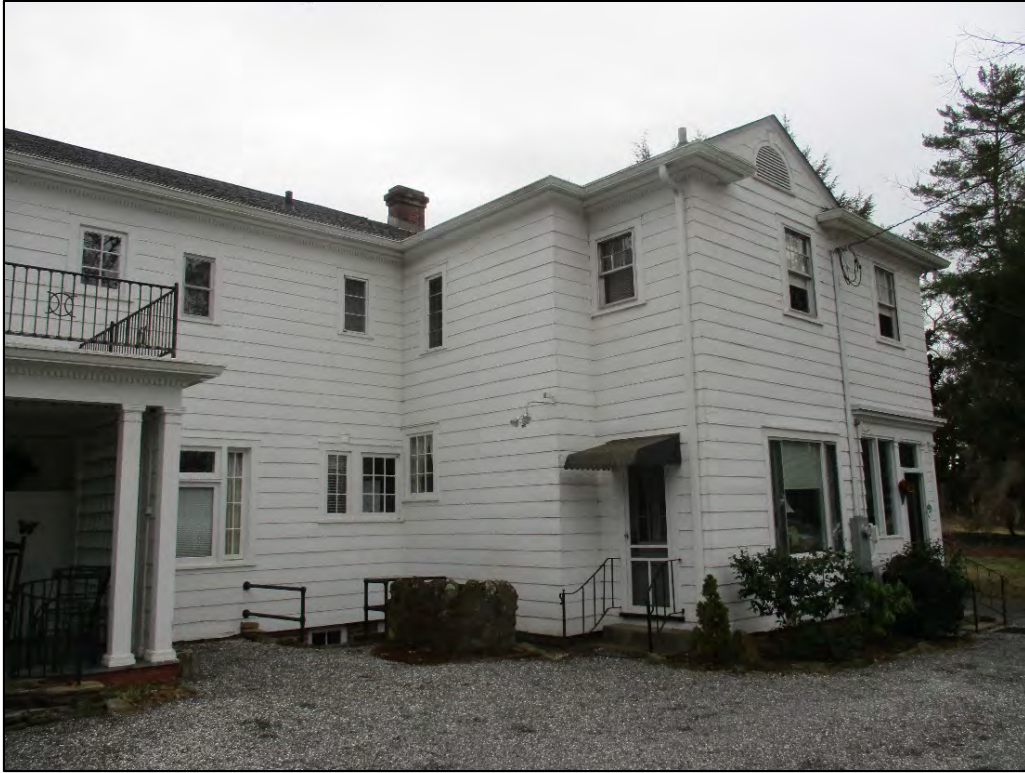
Rhodes House rear (west) elevation, view to the southeast
