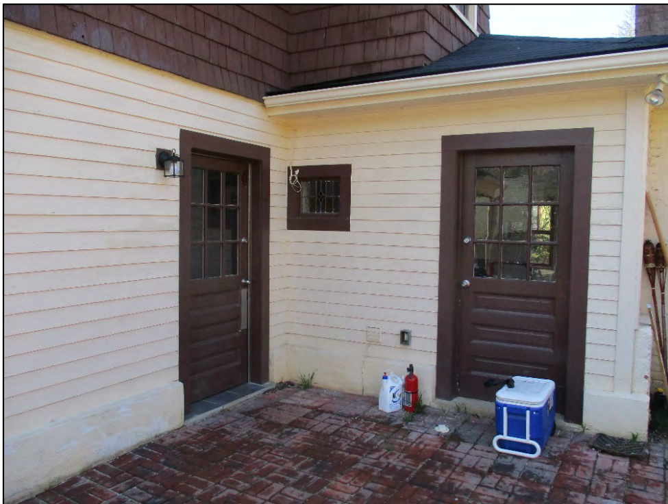
Martha Sayre House rear (north) elevation patio door and window detail
