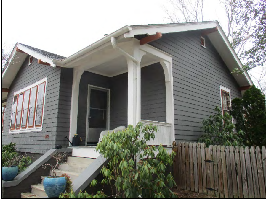
Oblique view of the façade and north elevation, view to the southwest
