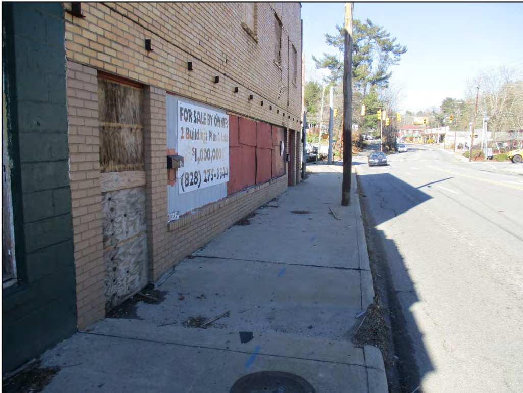
Former Moser Plumbing Building, view to the north along Merrimon Avenue along façade and sidewalk
