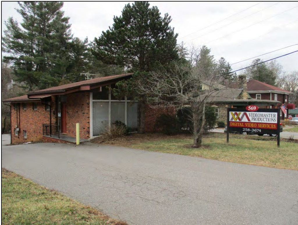
Ray Dental Office oblique view of the façade and north elevation, looking southeast
