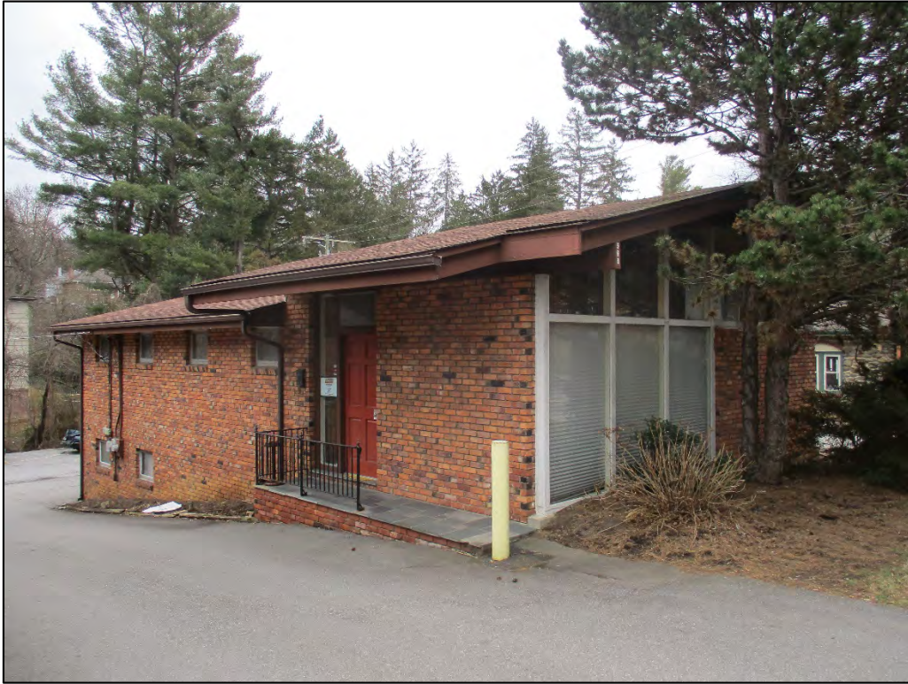
Ray Dental Office oblique view of façade and north elevation, looking southeast
