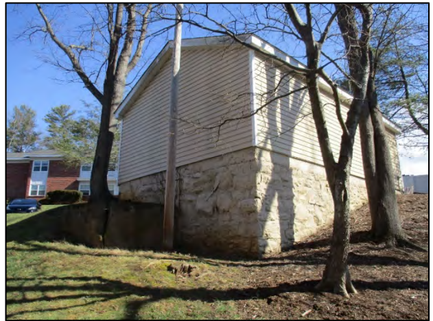
Edgewood Knoll Apartments outbuilding/garage, view to the northeast
