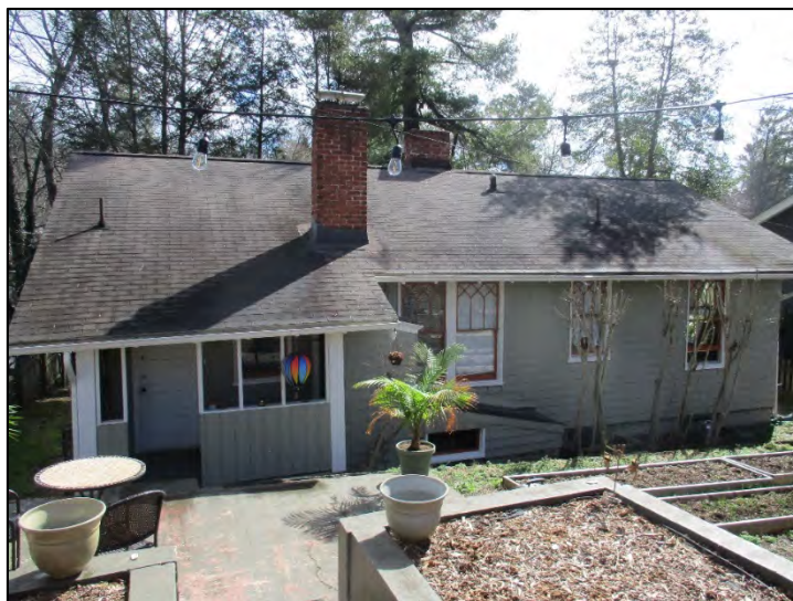
Lauerhass House west elevation view to the east
