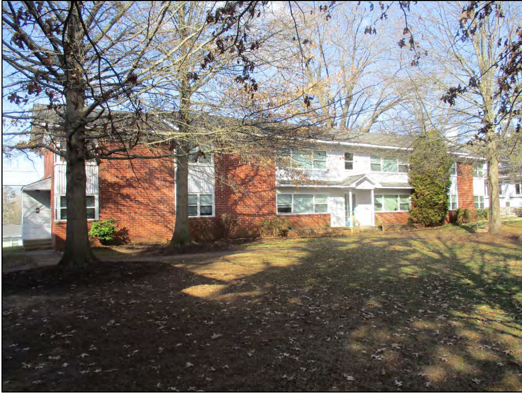
Edgewood Knoll Apartments Building 7 façade, view to northwest
