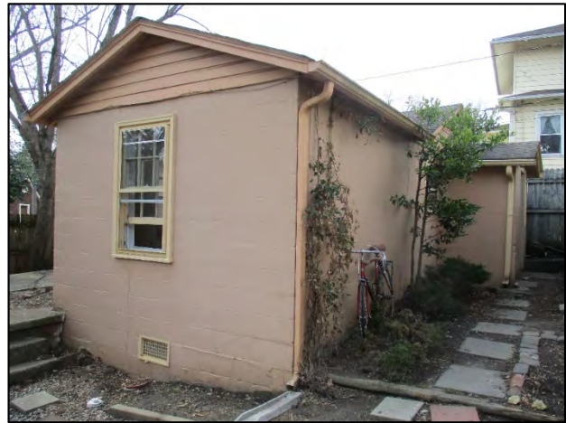
Lauerhass House outbuilding east and north elevation, view to the west
