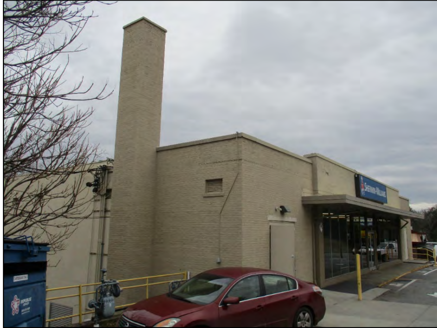
Burton and Son Furniture Store oblique view of portion of north elevation and façade, looking southeast
