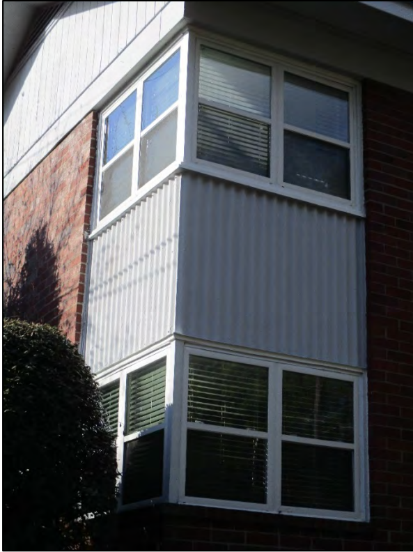
Edgewood Knoll Apartments Building 10 corner window detail, view to southwest
