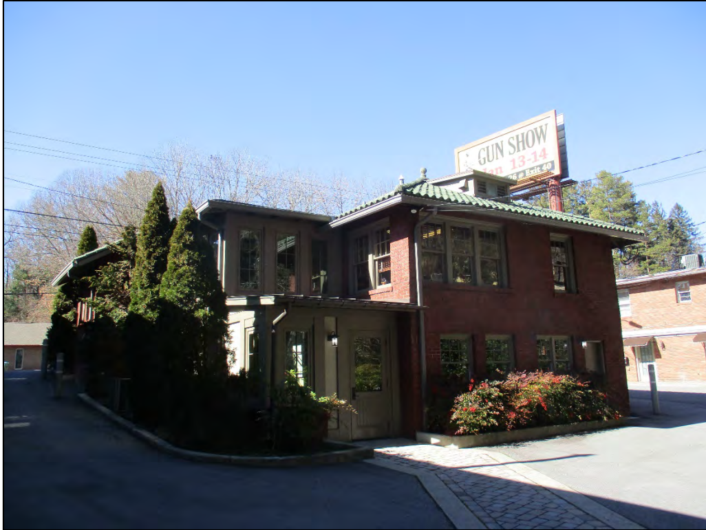
Chester W. Israel House rear (east) elevation, view to the northwest. Note non-historic addition in southeast corner of the house.
