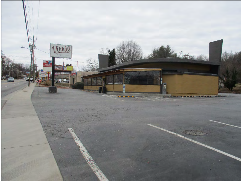
Former Athens Restaurant public façade, consisting of south and west elevation, view to northeast
