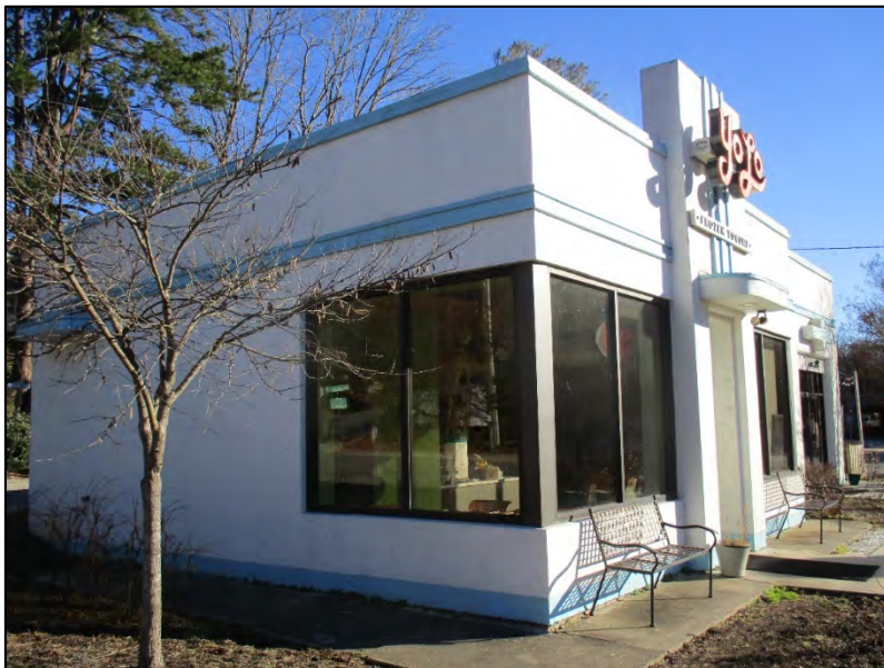
Former Woolsey Dip Amoco Station oblique view of the corner office and north elevation, view to the southeast
