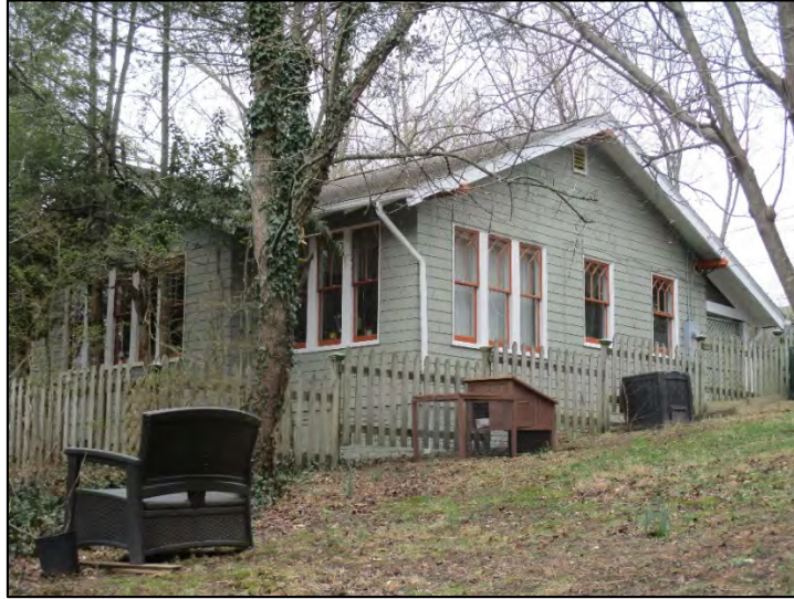
Lauerhass House north elevation view to the southwest
