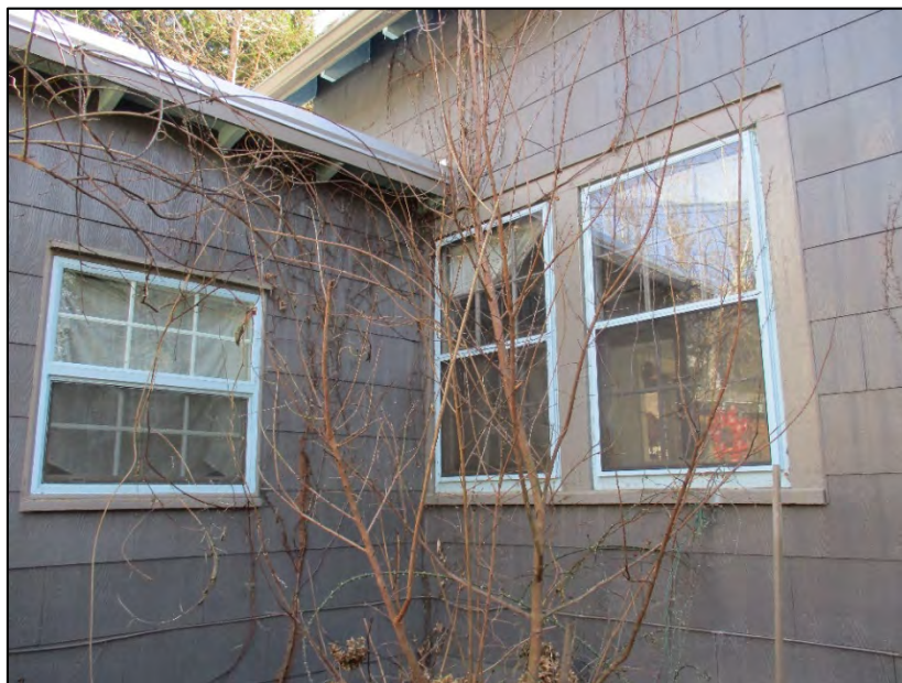
Weaver House north elevation windows, view to the southeast
