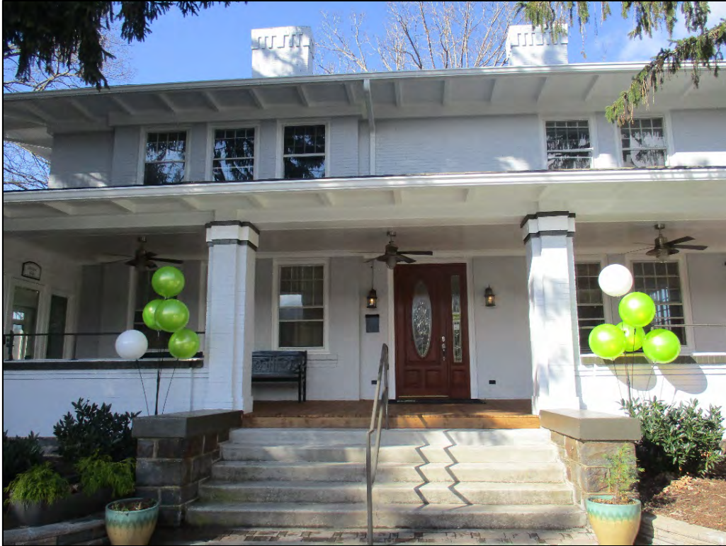
Edgewood Knoll Apartments leasing office front porch detail, view to west
