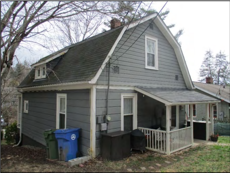
Joseph Lewis House west elevation, view to the southeast. Note the different German siding width in first and second stories.
