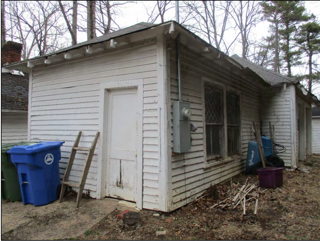
Rhoades House carriage house east elevation, view to the northwest
