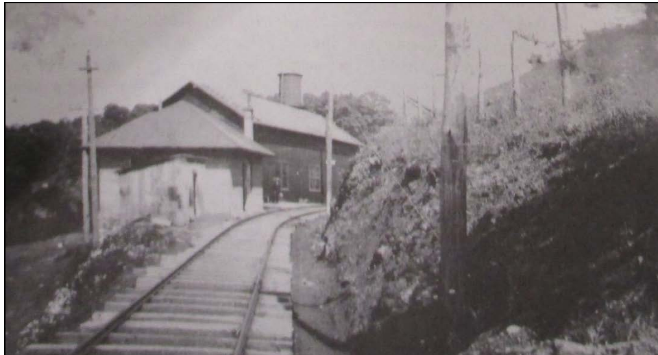
Exhibit 57. The Asheville & East Tennessee Newbridge Trolley Substation (BN1414) in foreground with car barn (no longer extant) behind. Source: Bailey et al, 2000: 64.
