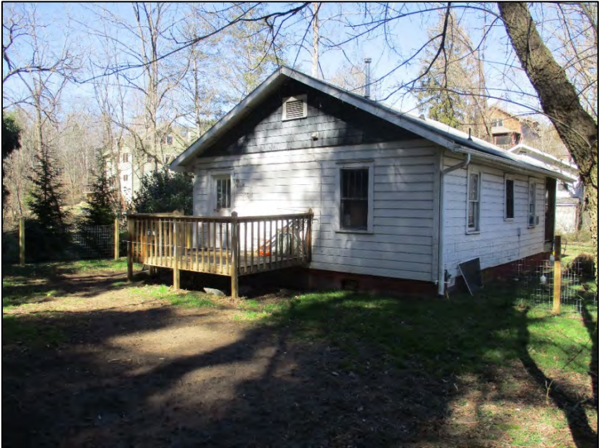
Atkins House oblique view of outbuilding south and east elevations, view to the northwest
