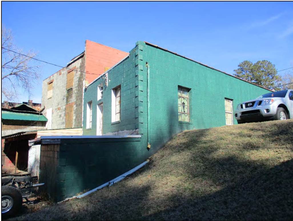
Former Keith's Super-Cleaners oblique view of the rear (west) and south elevations, looking northeast
