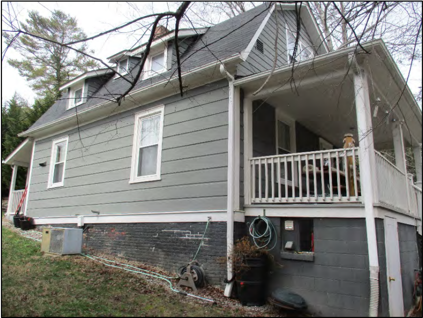
Joseph Lewis House south elevation, view to the north
