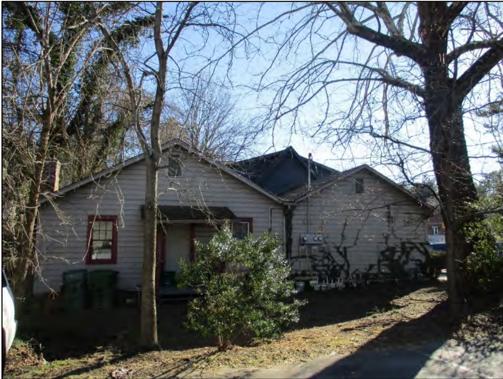
North elevation, view to south
