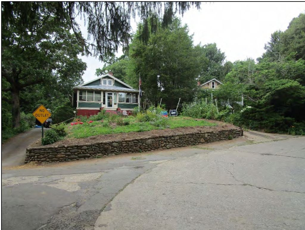
One and one-half story Craftsman bungalows, 144 Chatham Road (1925) at left and 148 Chatham Road (1923) at right
