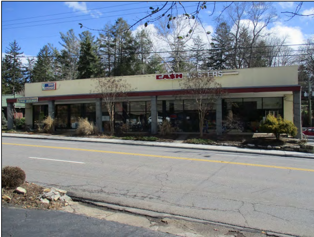
Former Morrison’s Furniture Store façade, view to northeast
