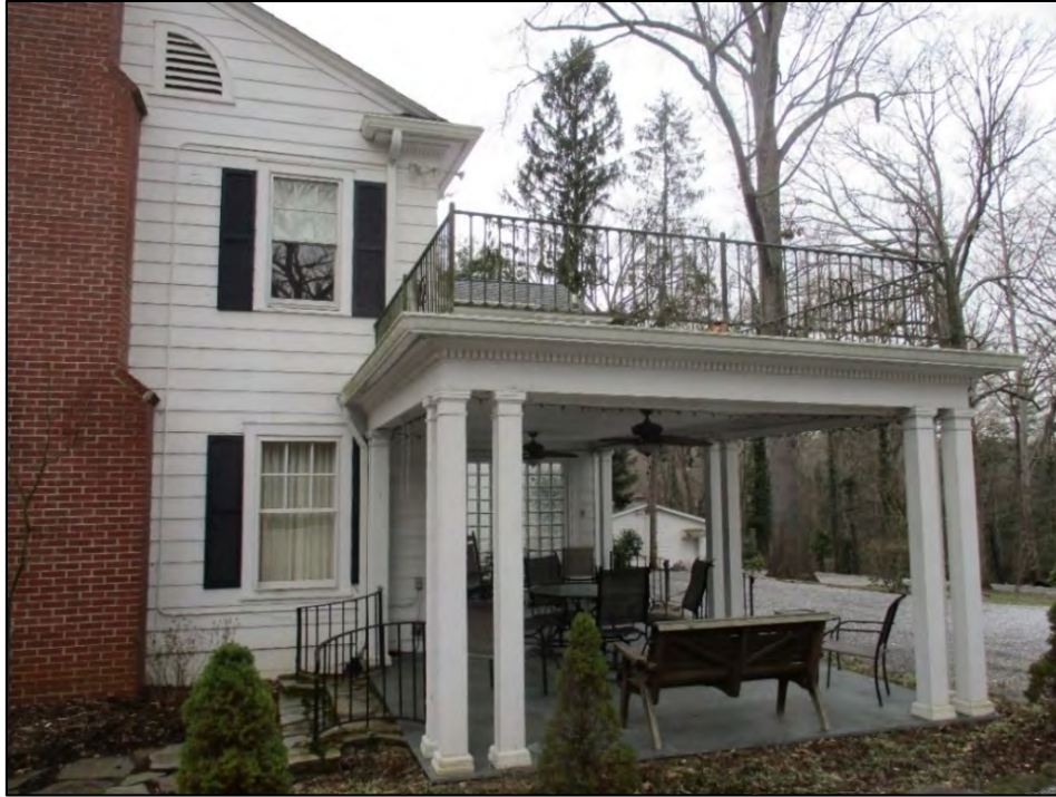
Rhoades House rear (west) elevation porch, view to the southwest
