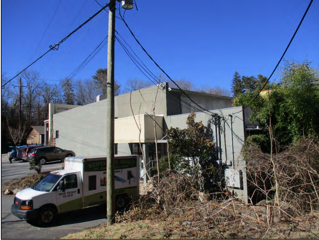
Former Morrison's Furniture Store south elevation, view to northwest
