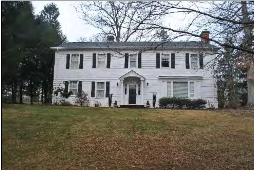
Rhoades House façade, view to the west
