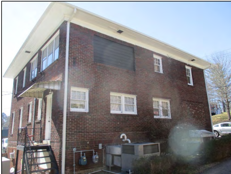
North elevation, view to the southwest
