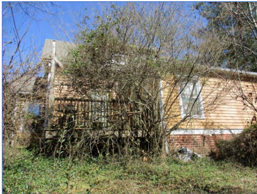
Guischarde House façade, view to the north of deck addition
