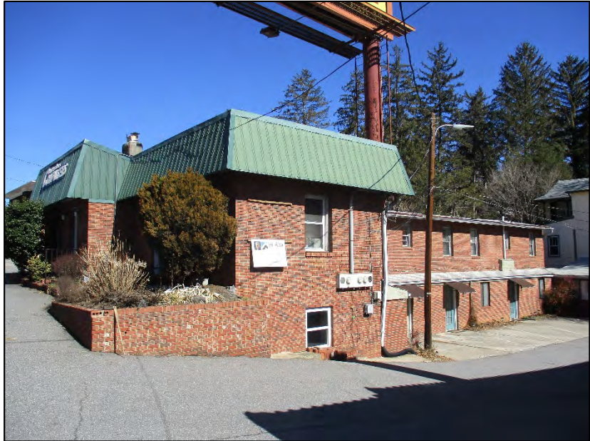
Farrwood Tourist Court oblique view of west and south elevations, view to the northeast
