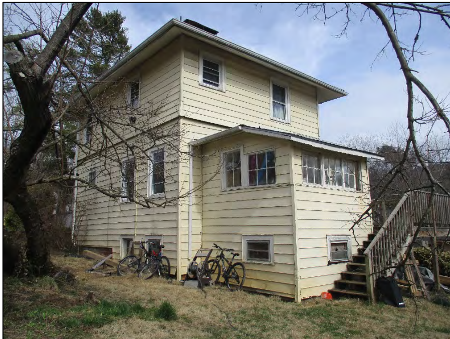
South elevation addition view to northeast
