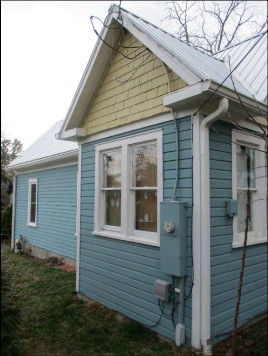
Barber House east elevation, view to southwest
