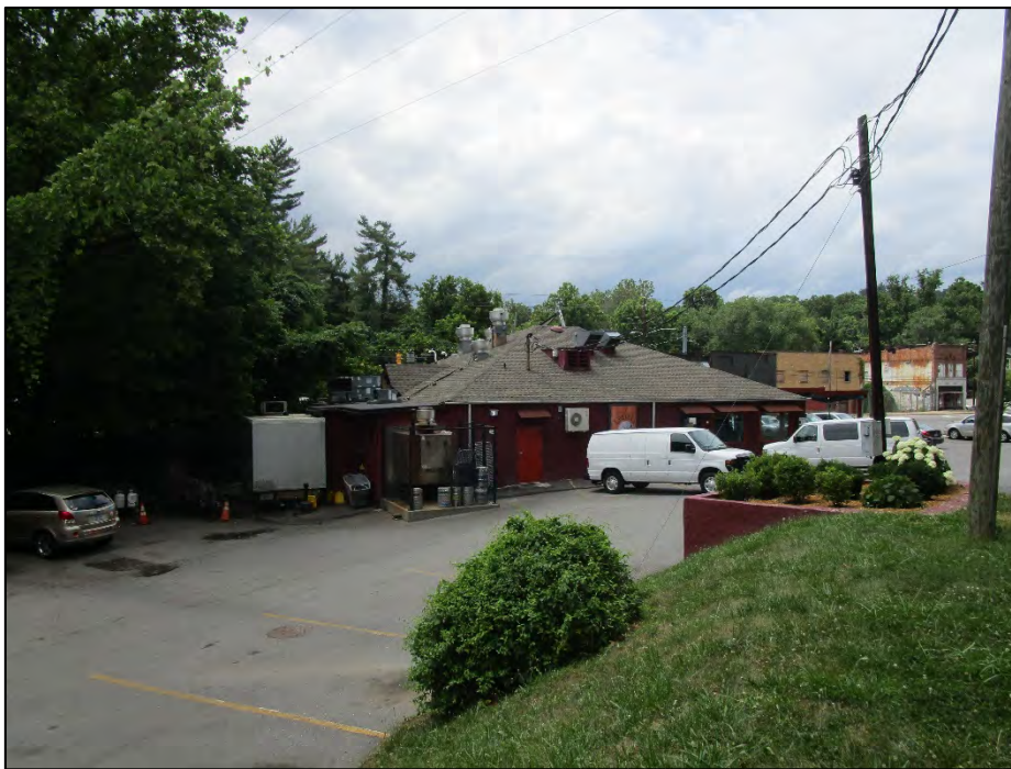
Former A&W Drive-In, oblique view of east and south (rear) elevations
