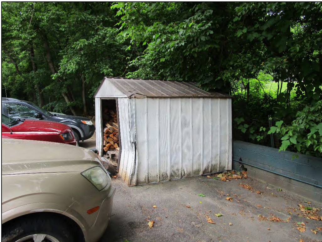
Former A&W Drive-In, aluminum wood shed south of the building. Concrete block walls are utilized in places adjacent to Reed Creek; the incised creek bank is located directly behind this wall.
