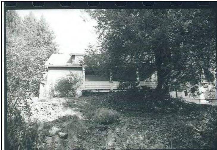
Exhibit 50. 7 Chatham, 1998 photograph from the BN3372 Historic Property Survey Summary
