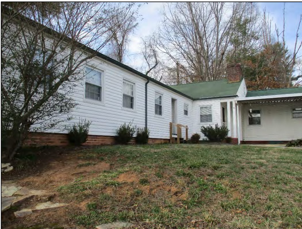
Clearview Terrace Apartments Building B, Unit 6 façade, view to north
