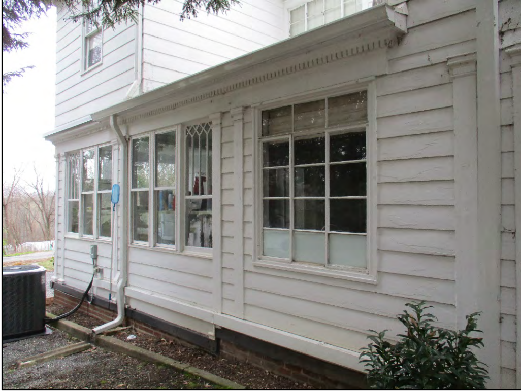
Rhoades House south elevation window detail, view to the northwest
