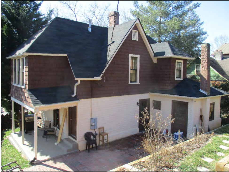
Martha Sayre House rear (north) elevation, view to the southwest
