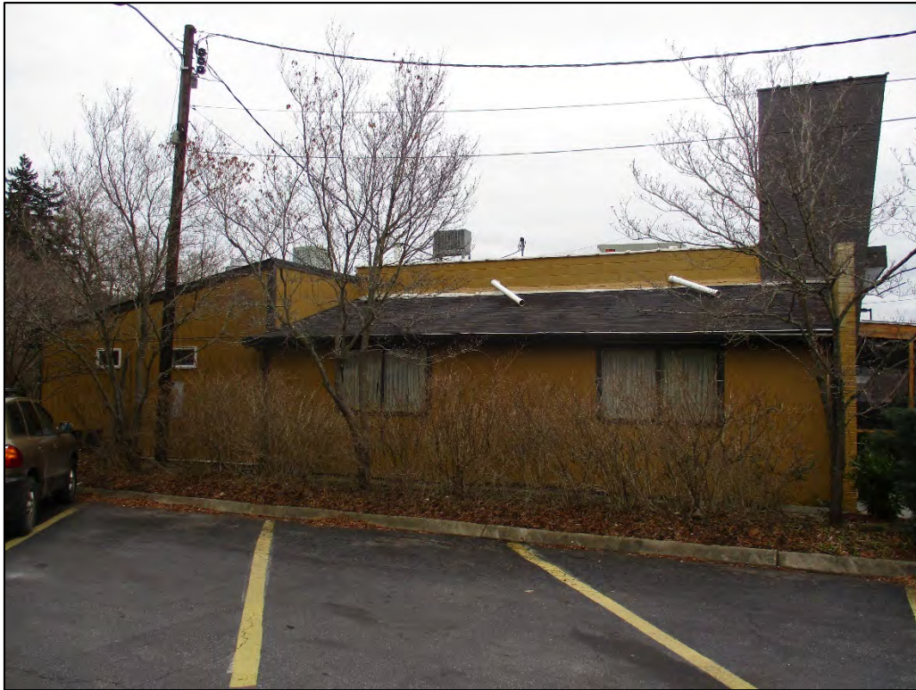
Former Athens Restaurant north elevation, looking south
