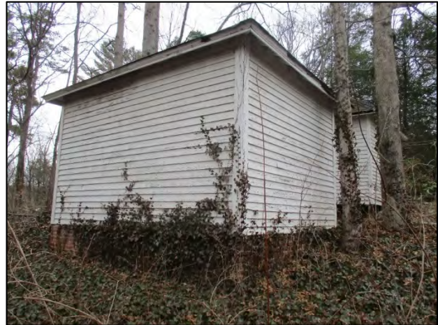
Rhoades House oblique view of Apple Shed south and west elevations, view to the northeast
