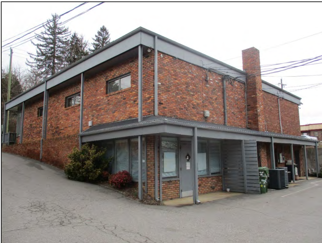
Thompson Building oblique view of the rear (east) and south elevations, looking northwest
