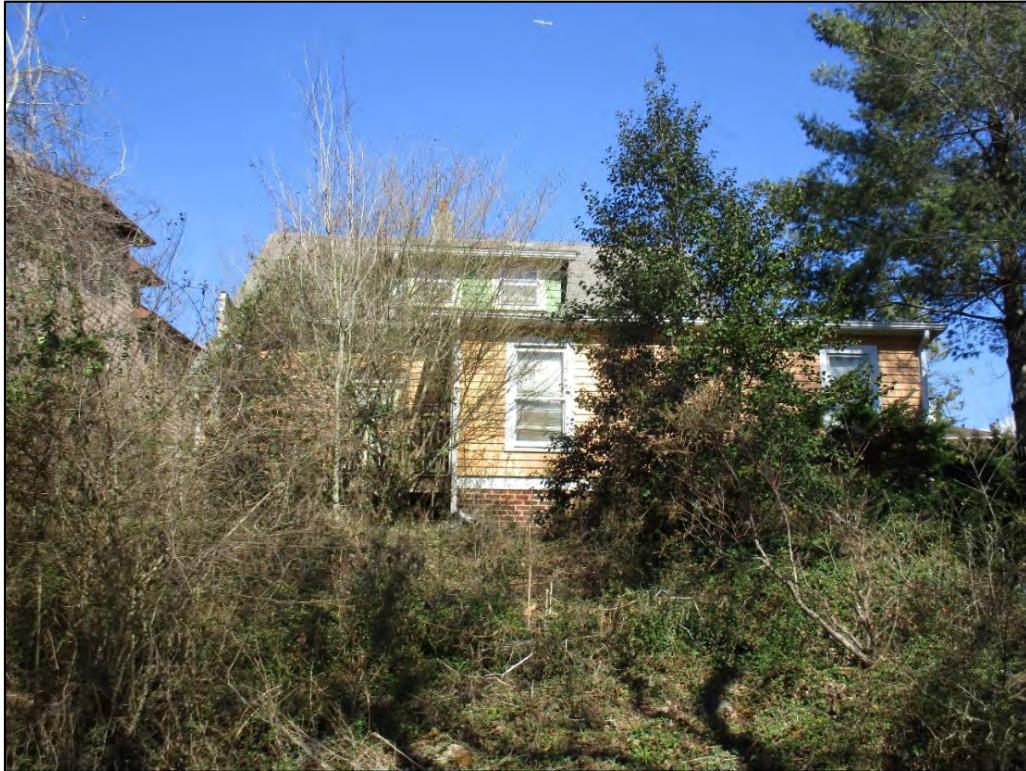
Guischarde House façade, view to the north
