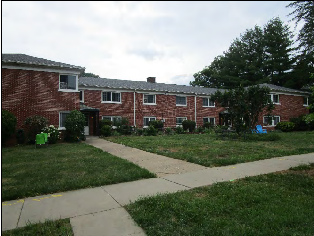
Exhibit 92. Kimberly Avenue Apartments (BN1174) (1951), 198 Kimberly Avenue in Kimberly Amendment to Grove Park Historic District
