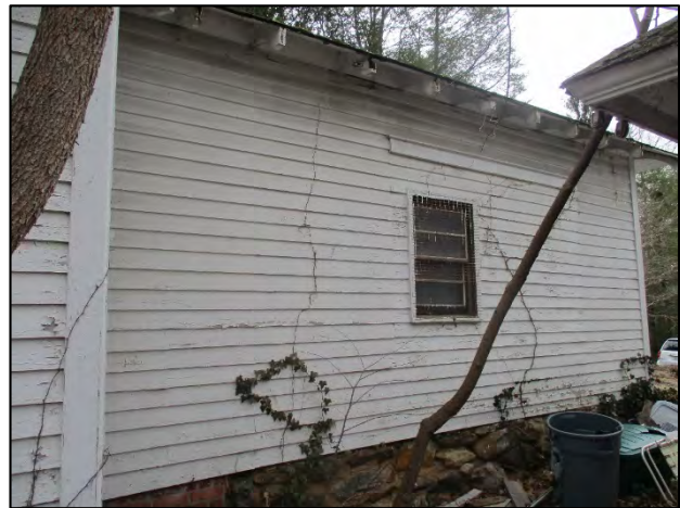
Rhoades House carriage house west elevation, view to the southeast
