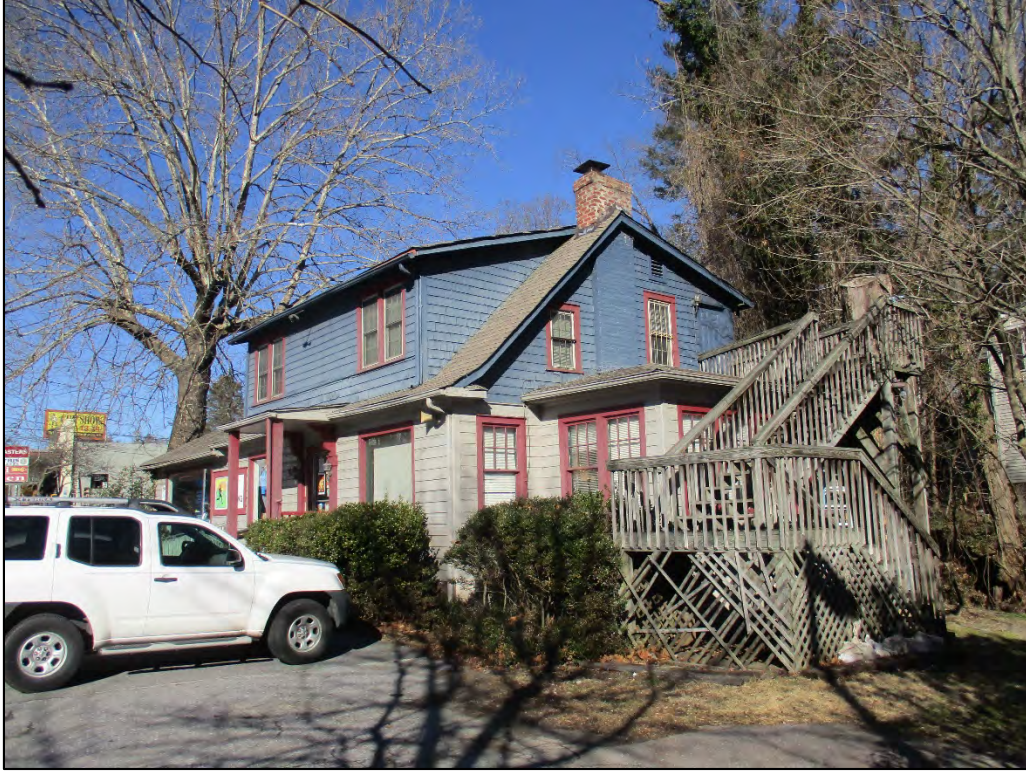
Oblique view of façade and south elevation, looking to the northeast
