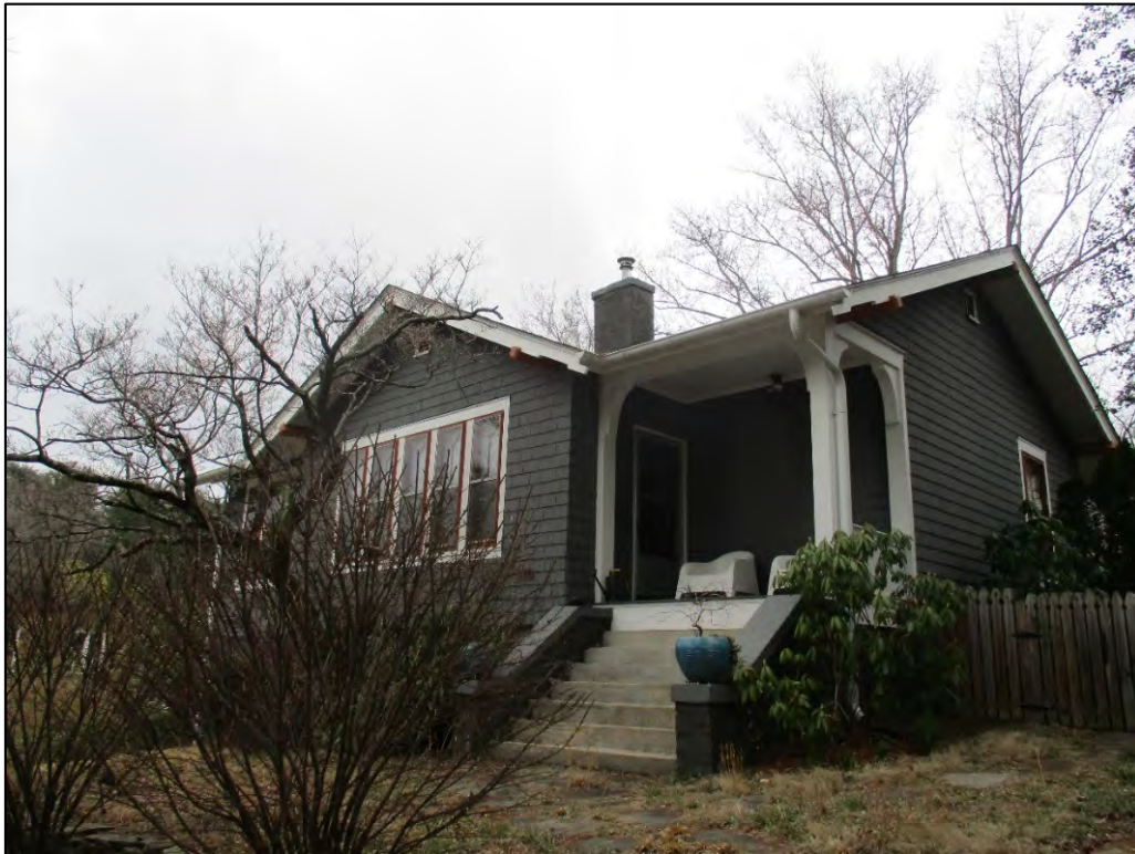
Façade, view to the southwest
