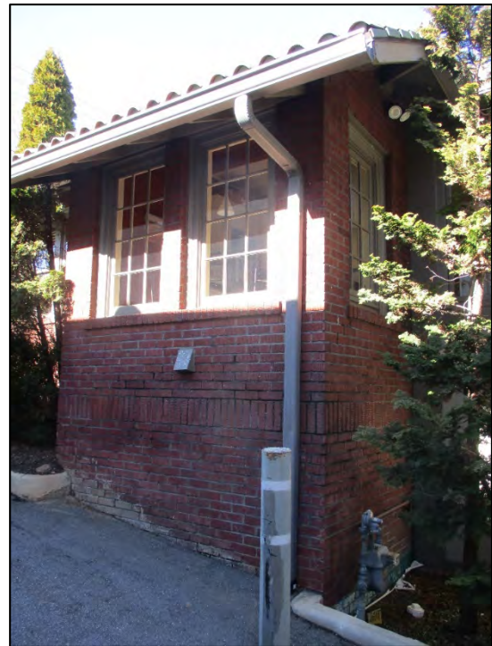
Chester W. Israel House south elevation shed wing detail, view to northwest
