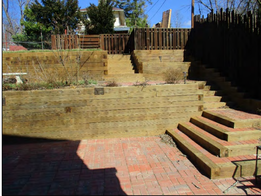
Martha Sayre House patio and backyard, view to the north
