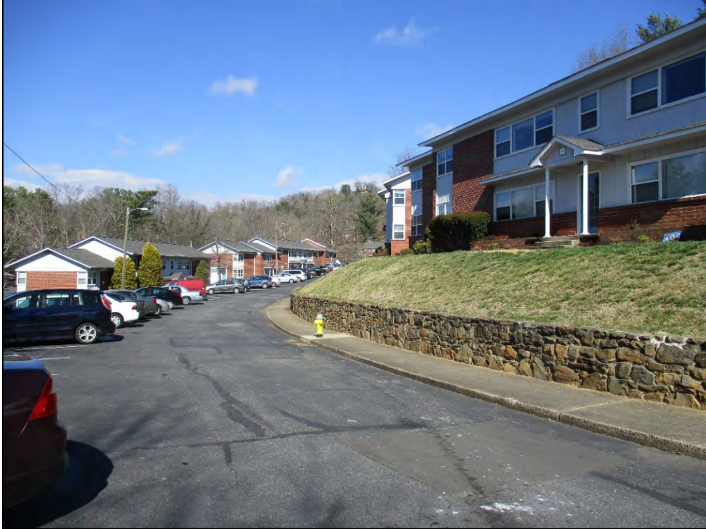
Edgewood Knoll Apartments, view to north of Edgewood Knoll Road streetscape, with stone retaining walls and sidewalks
