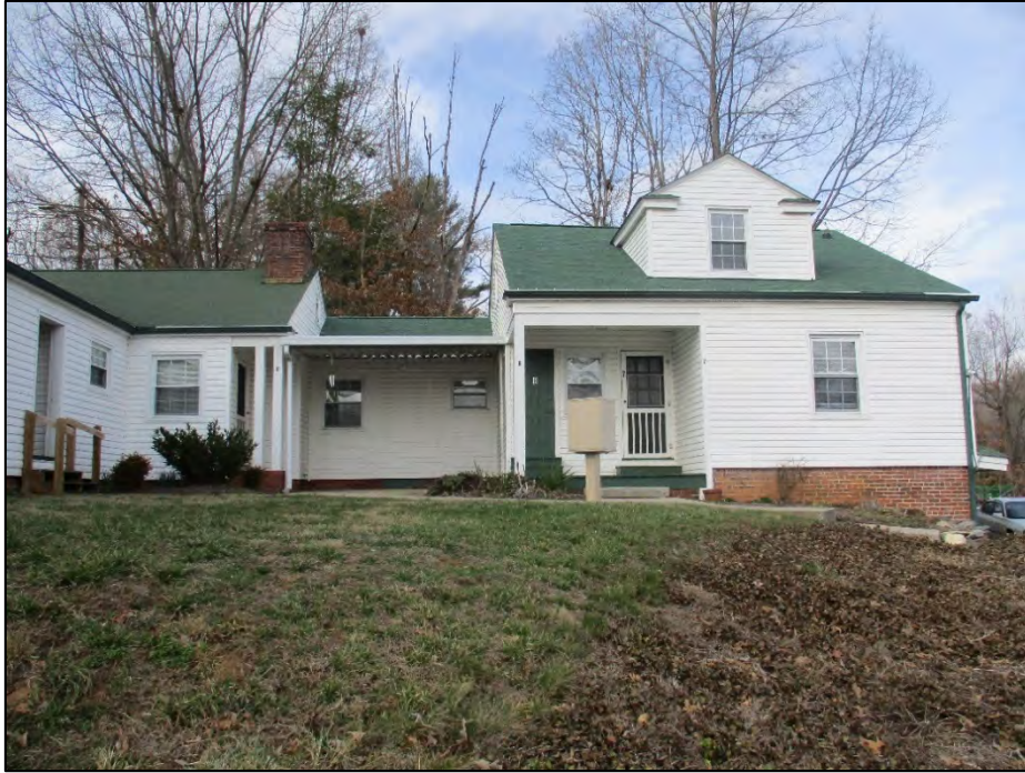
Clearview Terrace Apartments Building B, Units 6, 7, and 8 facade, view to north
