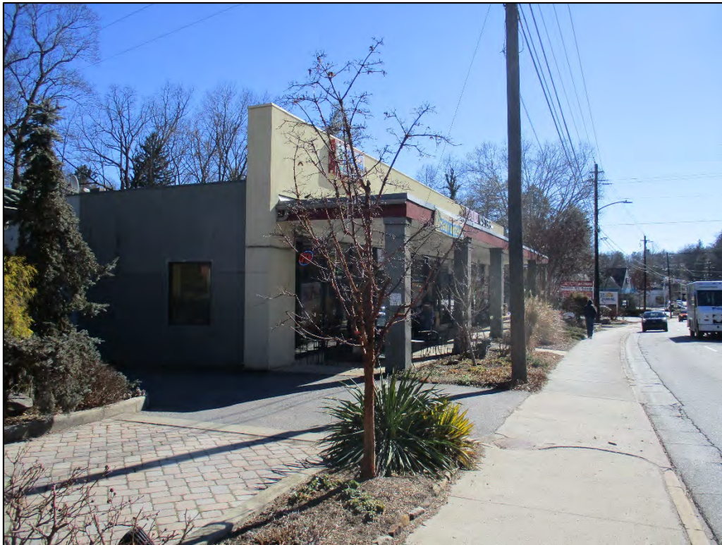
Former Morrison's Furniture Store, view south along Merrimon Avenue
