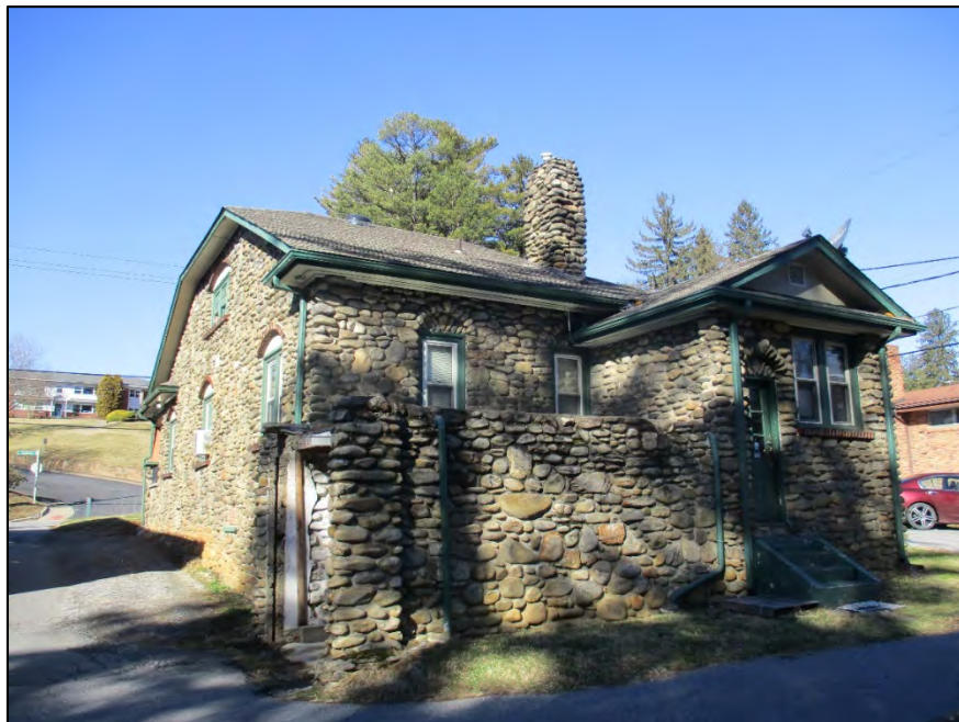
Former Belva L. Saunders House oblique view of east (rear) and south elevations, facing northwest. The garage is in foreground; the Ray Dental Office Building is visible at right.
