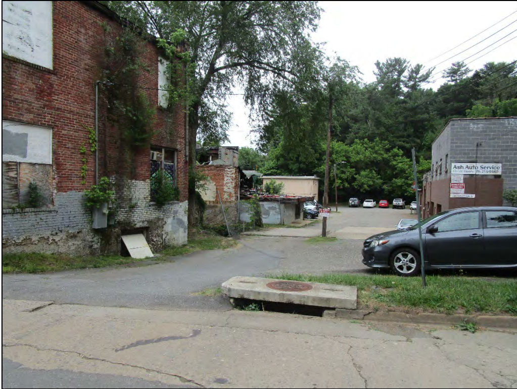
Woolsey Dip Historic District, view to the south from Chatham Road of the alley
