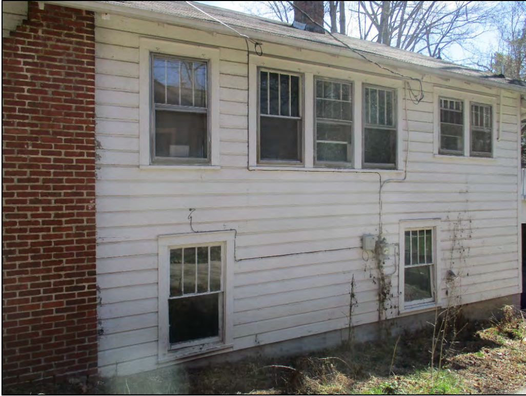
Atkins House west elevation, view to the southeast
