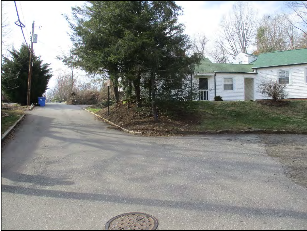
Clearview Terrace Apartments Building A, Unit 1 façade, view to west along Clearview Terrace
