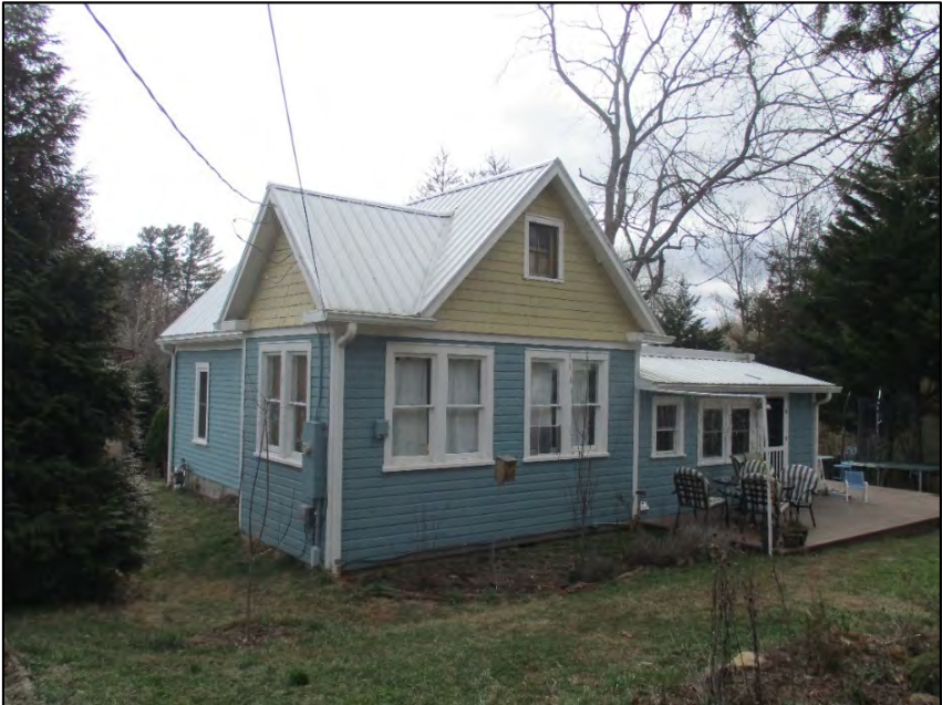
Barber House north elevation, view to southwest
