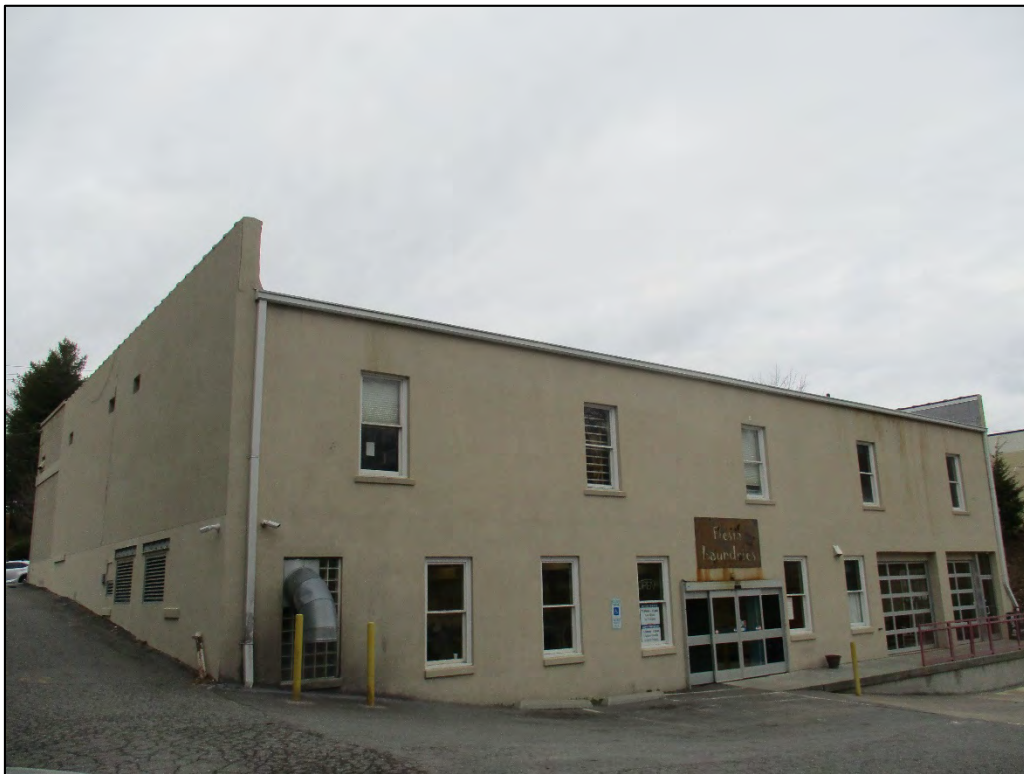
Burton and Son Furniture Store oblique view of rear (east) elevation and south elevation, looking northwest
